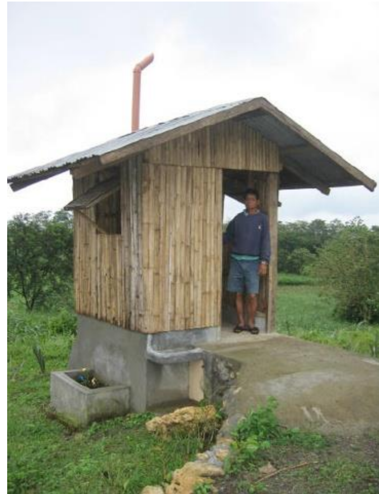
Exterior views of Double-Vault UDDTs, Philippines
