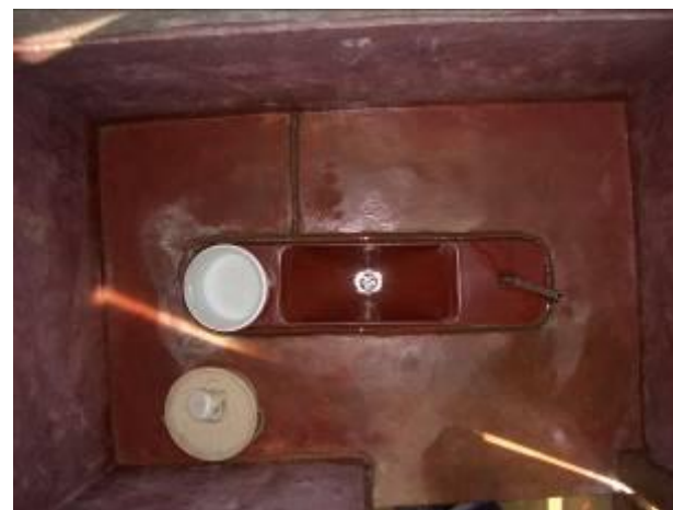
Exterior and interior view of Double-Vault UDDT by Practical Action, Sri Lanka
