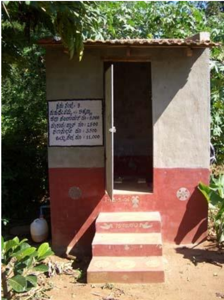
Exterior and interior view of Double-Vault UDDT by Rural Dev. Dep. Karnataka State, India
