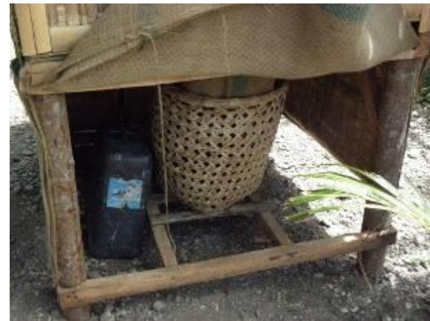
Low-cost UDDTs at coastal area in Libertad Municipality, Philippines
