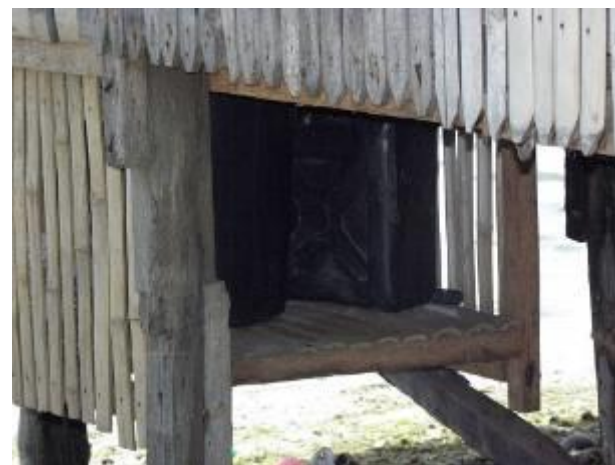
“Hanging UDDTs” at coastal area in Libertad Municipality, Philippines
