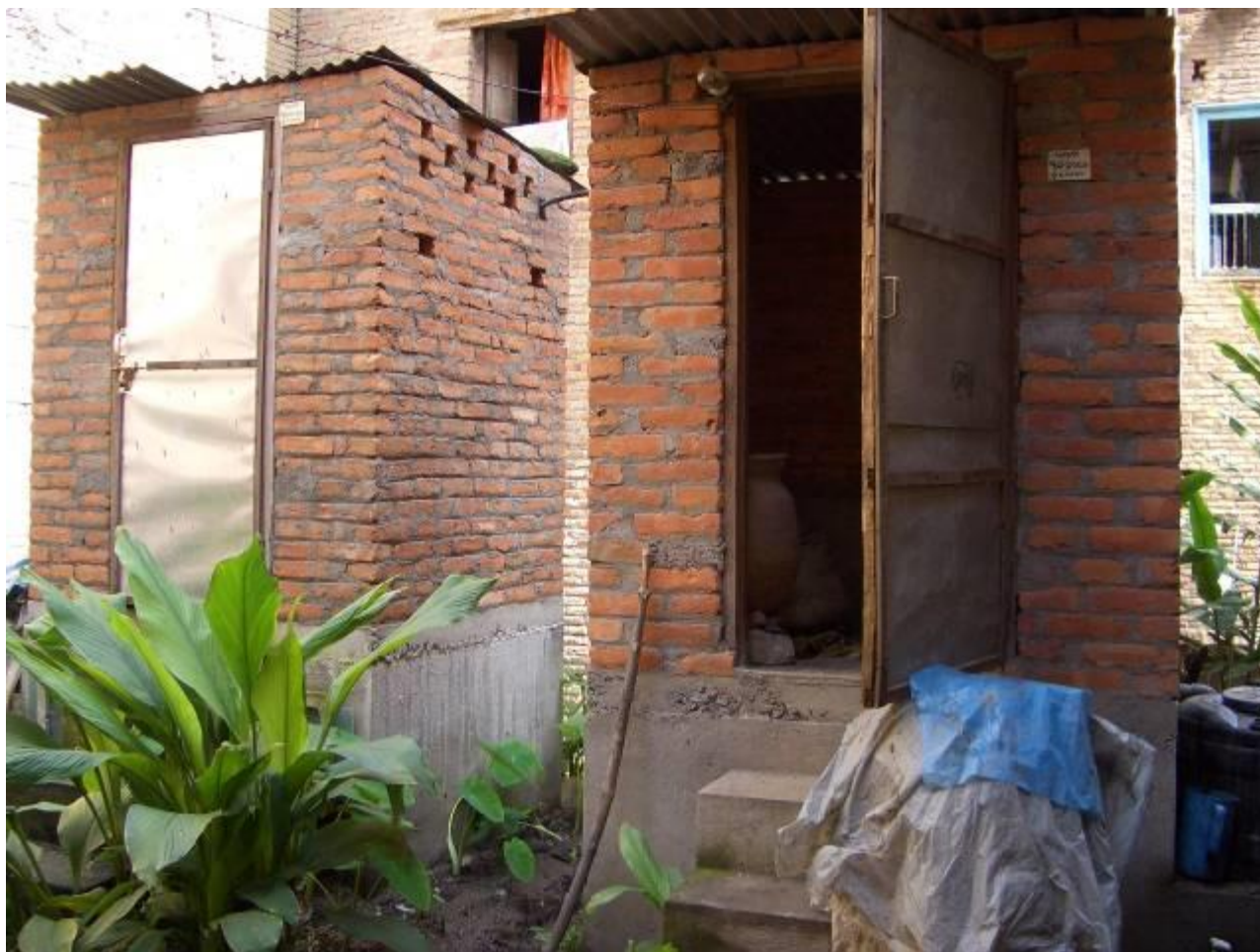
Exterior view of Double-Vault UDDTs by ENPHO, Nepal
