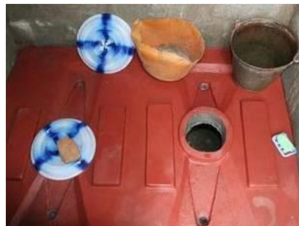
Exterior and interior view of Double-Vault UDDT by SCOPE, India
