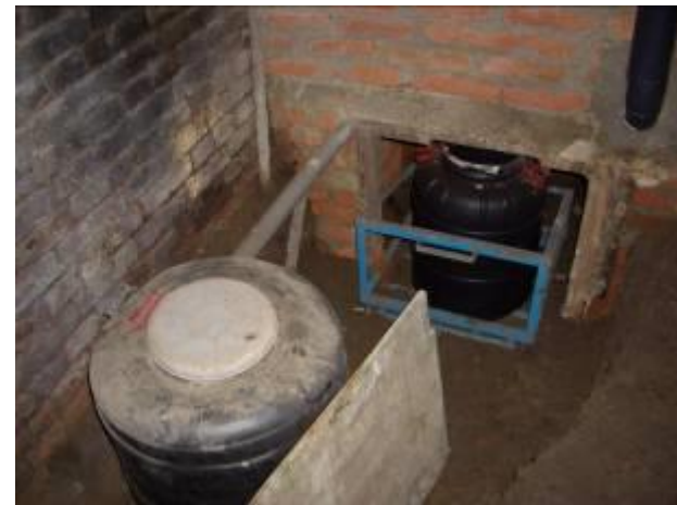
Single-Vault UDDT at ground floor level of multi-storey building, Kathmandu, Nepal
