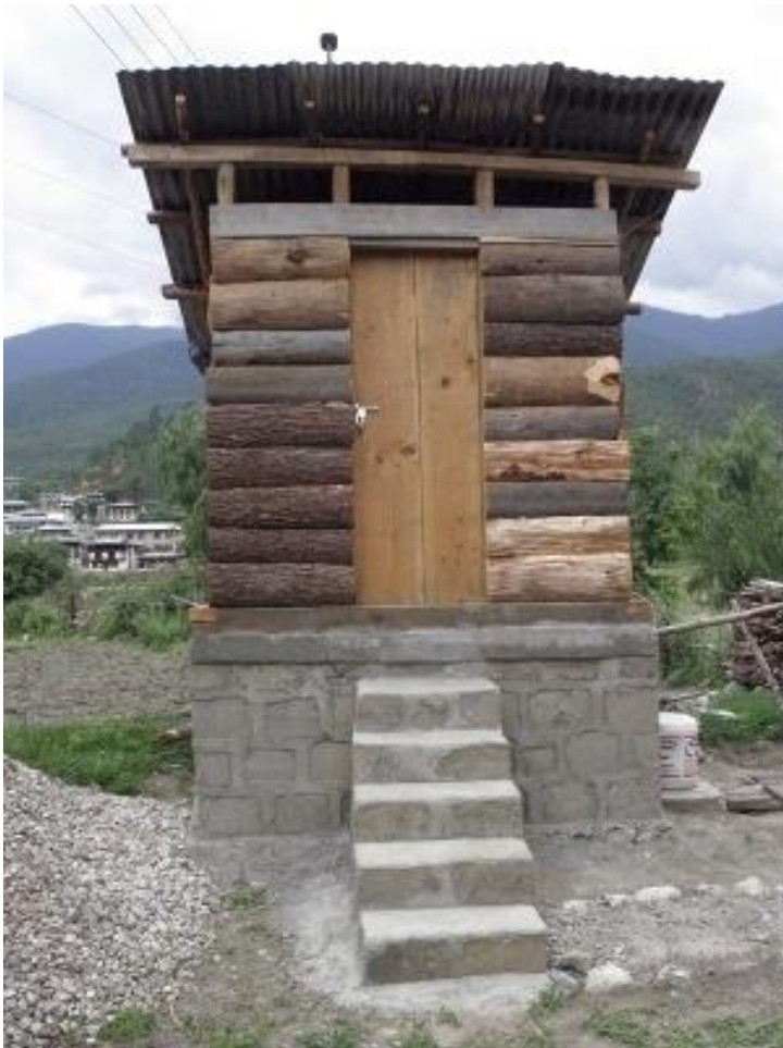
Exterior and interior view of Double-Vault UDDT by Ministry of Health, Bhutan
