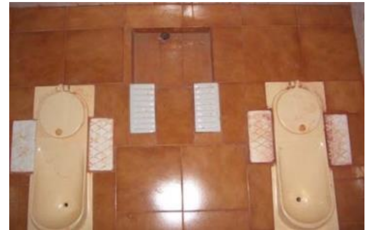
Interior view of Double-Vault UDDTs
