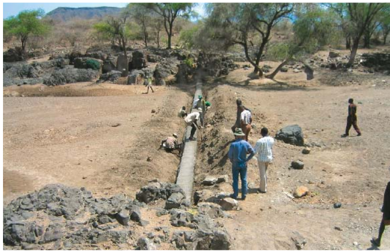
Dam under construction
