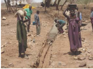
Construction of topcover
