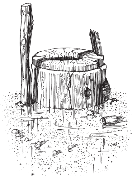
Figure 15.3. A damaged well, showing cracks in the walls
