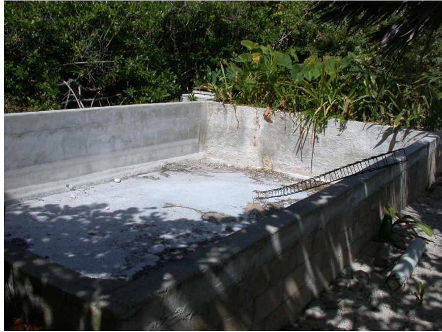
Figure 3: An unfinished constructed wetland built using concrete blocks
