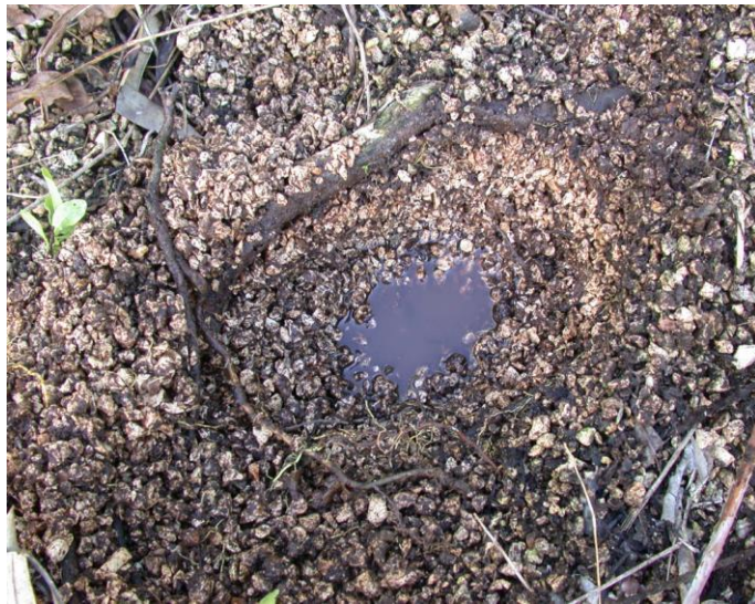
Figure 6: Smaller aggregate at Las Casitas wetland. The aggregate has been removed to expose water just a few centimeters below the surface.
