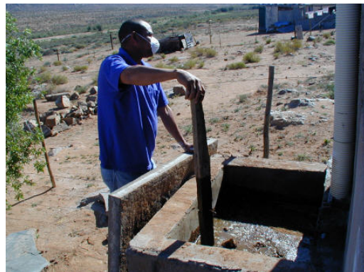
Appendix figure 5: Unhygienic emptying of a VIDP. Urine does not flow out because the soil is not permeable enough
