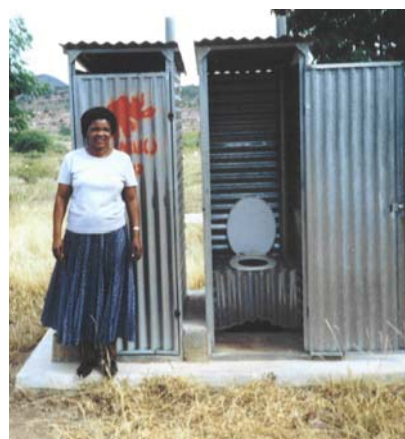
Figure 4: common appearance of a pit latrine (two top structures over one pit is rare in the village).
