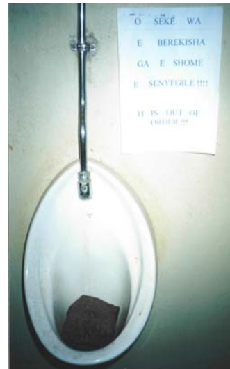
Figure 16: Unused urinary in the church. A stone was put in to emphasise it should not be used. By using a pit latrine, scarce water can be saved (Sekwati, 2002)
