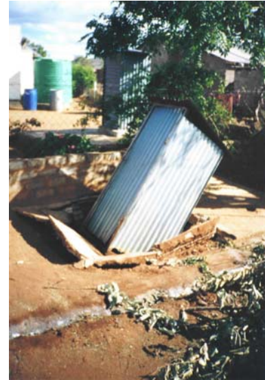
Figure 19: One evening I arrived in Mhlaletse village. A son of the priest had an embarrassing accident. While he was sitting on the toilet the top-structure of the (simple) pit latrine collapsed. Accidents like these are not rare in the village.
