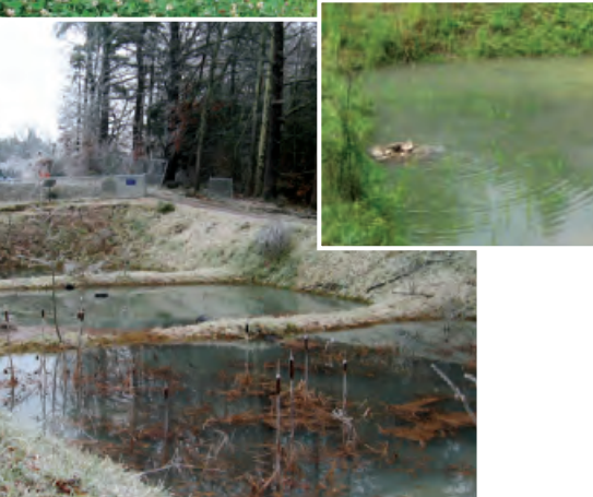
Subsurface gravel wetlands do an exceptional job of treating stormwater quality and managing water quantity. The design for the gravel wetland pictured above is helping New Hampshire's Department of Transportation meet Total Maximum Daily Load (TMDL) standards for numerous transportation improvement projects.
