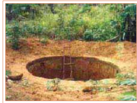
Pit for the tank construction
