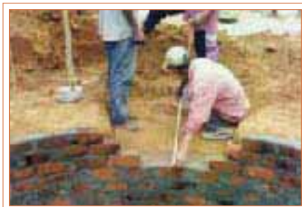
Measurement taken for the inlet construction
