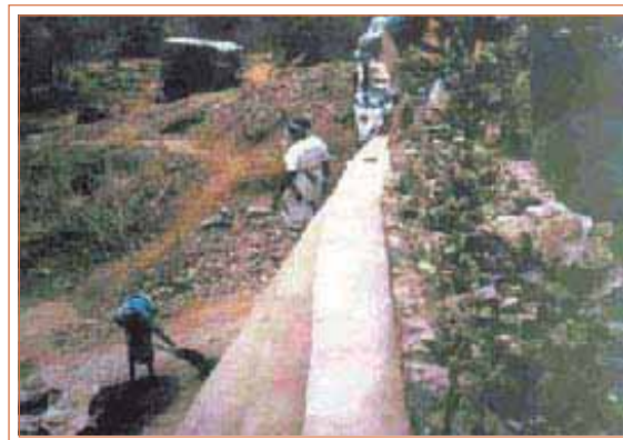
Women as local scale water managers: rock catchment construction in Kenya (Gnadlinger)
