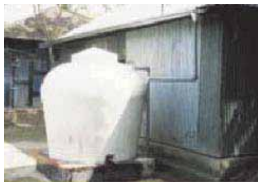
Bangladesh: Pottery storage (MOTKA) for rainwater; ferrocement tank storage
