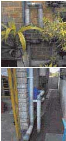
First-rain separator - Segregator: Simple and easy to maintain
