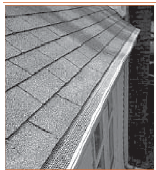
One example of a flat screen over the gutter to keep large debris out of the tank. A problem with gutter screens is that they require a lot of maintenance to keep leaves and debris from piling up and blocking the screens. Also, dirt on the leaves can still be washed into the storage tank.
