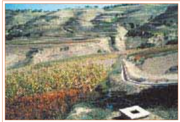
The rainwater is collected from asphalt paved highway and conveyed to underground water cellars through a concrete lined ditch
