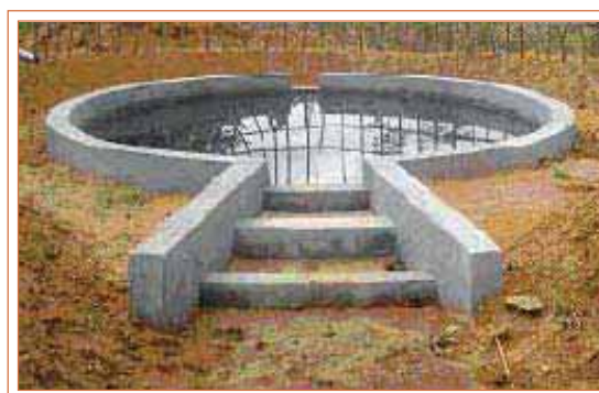
After the completion of the rainwater harvesting tank
