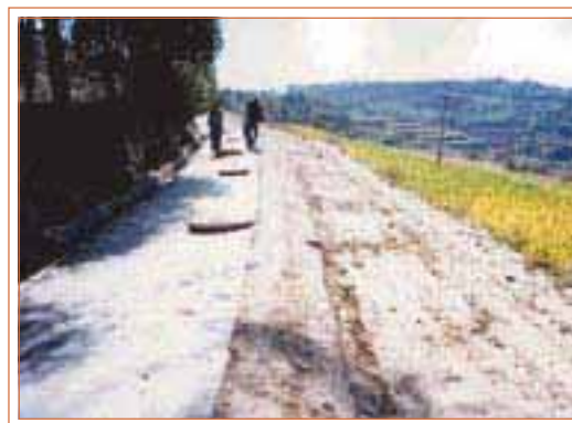
A group of water cellars fed with rainwater collected from concrete lined sports yard of a primary school
