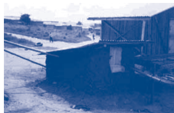
Completed tank (Pictures: D. Rees)
