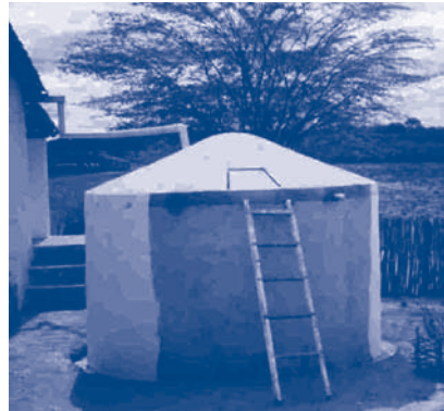
Finished tank being painted
