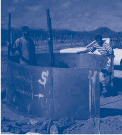
Screwing together the steel sheet form
