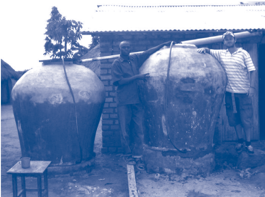
1,600 litre mortar rain-jars transported to site by handcart and installed in cascade. The right hand jar gives washing water and the left-hand jar gives potable water. Note the narrow (50 mm) guttering and the cheap hosepipe used instead of a tap.
