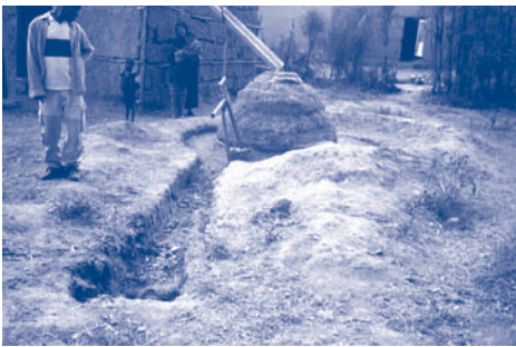
Thatched tank in Ethiopia Note: drainage to pit
