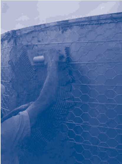
Application of the first layer of mortar on top of the wiring
