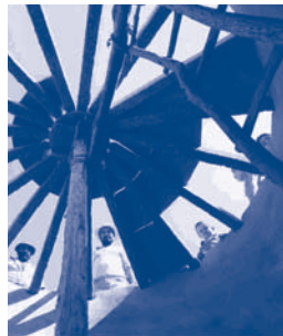
Installing the roof
