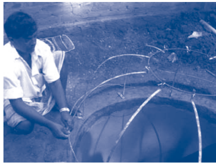
Fixing the frame for the dome
