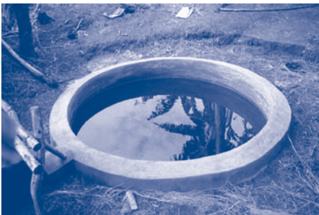
Underground tank with sloped ring beam
