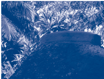
Detail of access to tank
