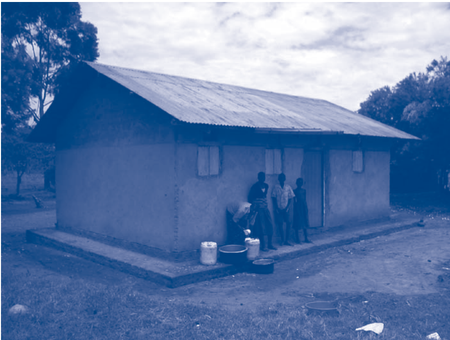
Figure 1.2. Informal roofwater harvesting (Picture: T.H. Thomas)
