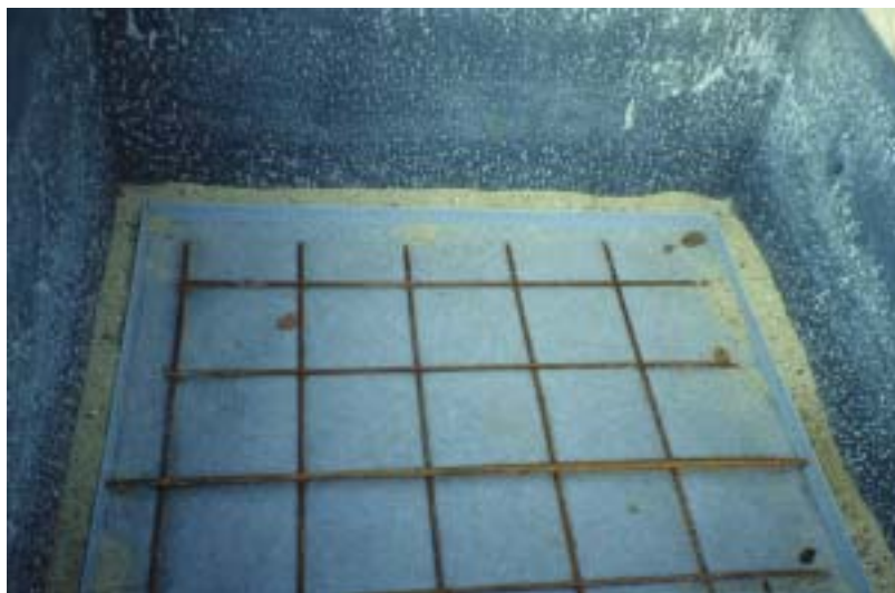
Plate 4.18: Surface mat installed onto a SSF bed at Surbiton (London, UK)
