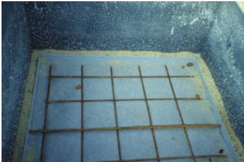
Plate 4.7: Surface Mat Installed onto a SSF Bed at Surbiton (London, UK)
