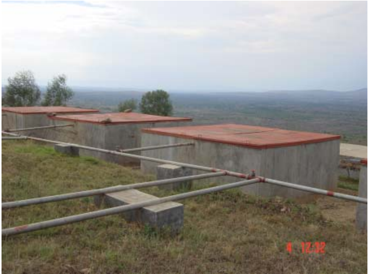
Plate Error! Style not defined..Error! Bookmark not defined.: Covered community scale SSFs at Nyabwishongwezi Water Treatment Plant, Umatara, Rwanda
