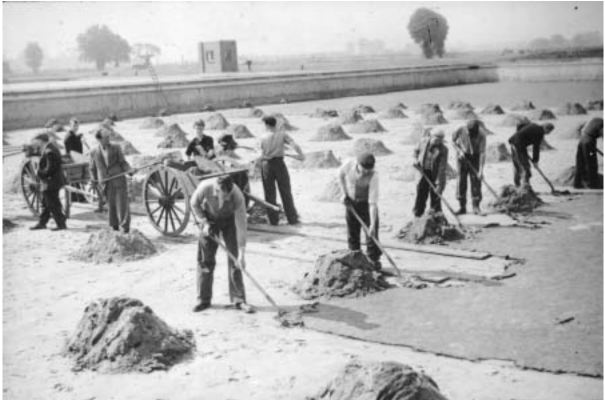
Plate 5.1: Manually skimming a SSF at the Walton treatment works in the 1940s, London (UK)
