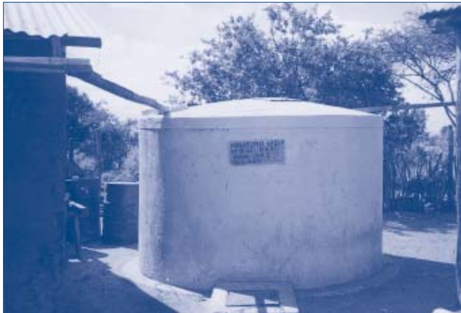
Fig. 7.1. Simple roof catchment and storage
