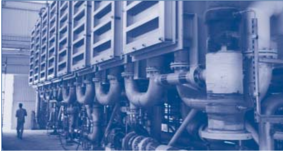
Fig. 18.2. Multi-effect distillation plant with vapour compression (MED +VC) in Mindelo, Cape Verde (capacity: 2400m 3 /day) (photograph by Jan C. Schippers)
