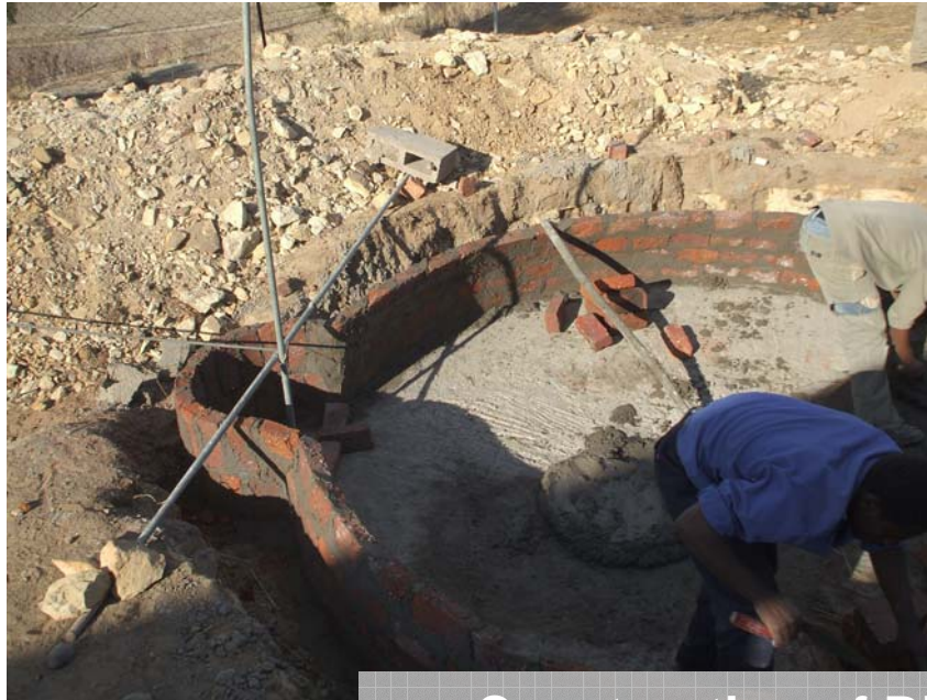
Construction of Biogas plants
