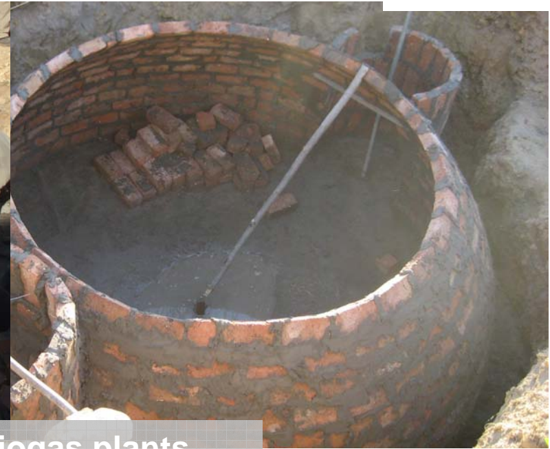
Construction of Biogas plants
