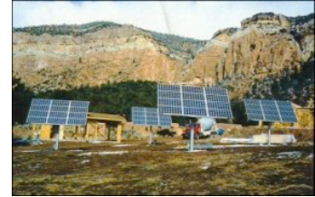
PV panels mounted on “tracking” arrays follow the sun like flowers.
