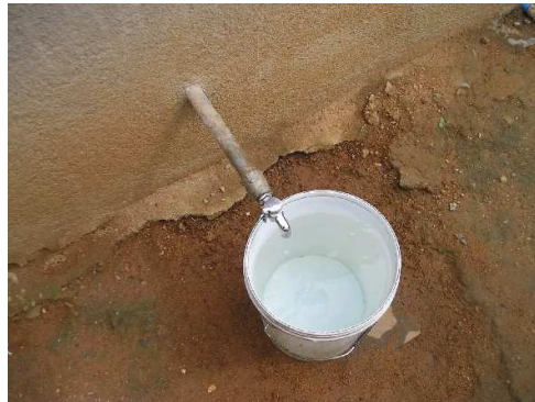
Fig 18: Clear water from a well kept rainwater harvesting system
