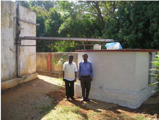
Fig 9 & 10: A good first rain separator with end cap on the wall Gate valve can also be used
