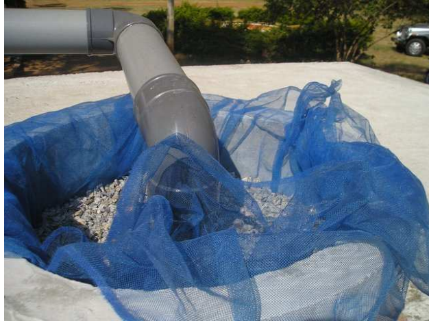
Fig 11: A good filter with mesh and gravel on top
