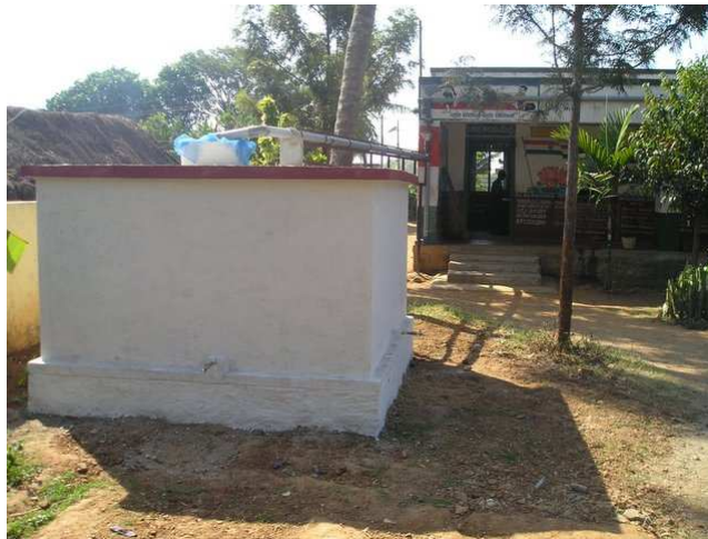
Fig 12: A clean storage tank on a platform painted white on the outside
