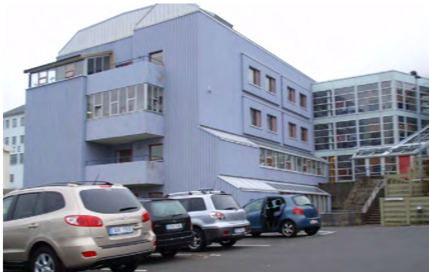
Figure 3. Klaksvik Hospital. The sewage line was accessed through a manhole at the parking lot
