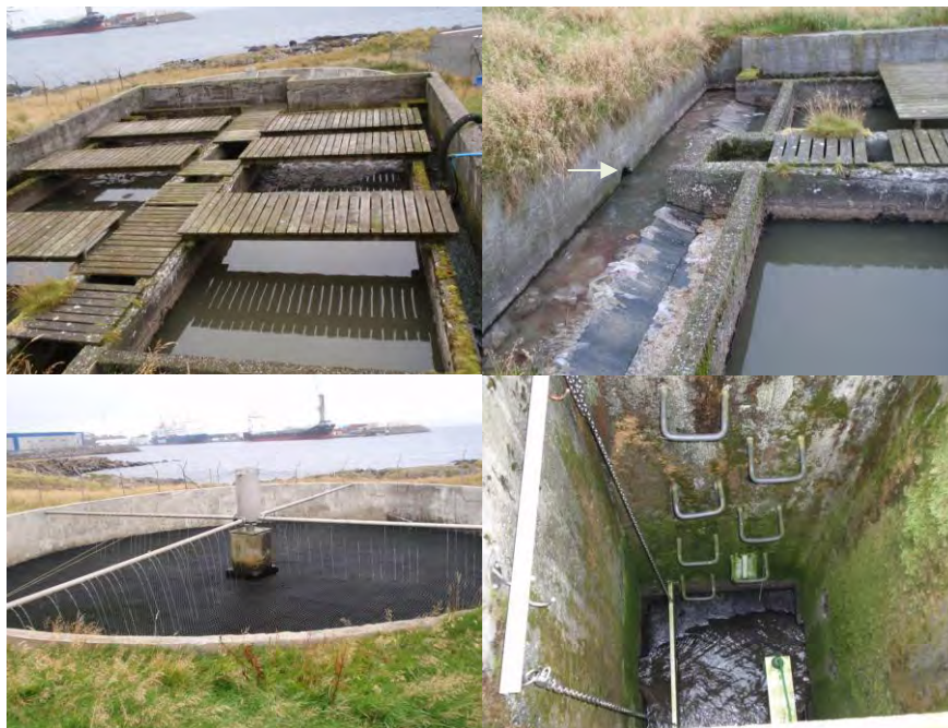
Figure 2. The Main Hospital (Faroe Islands) WWTP
