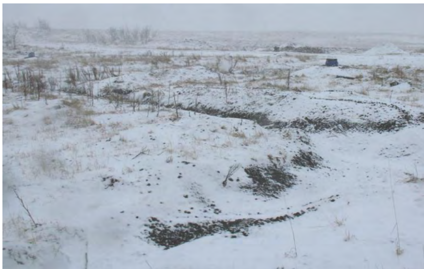
Figure 6. The snow-covered gravel bed outside the Hveragerði WWTP where the canals are periodically flooded and sludge accumulates
