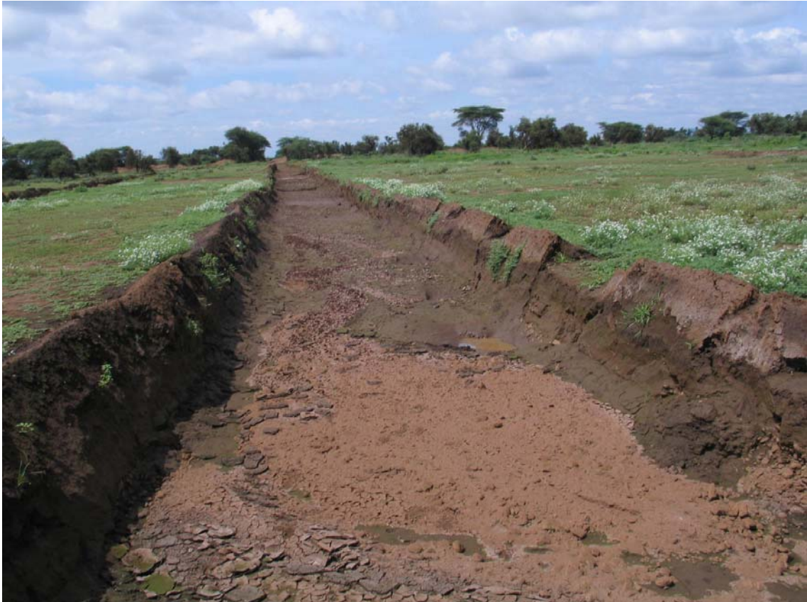
Figure 4.2 Siltation at the bottom of the contour trench.
