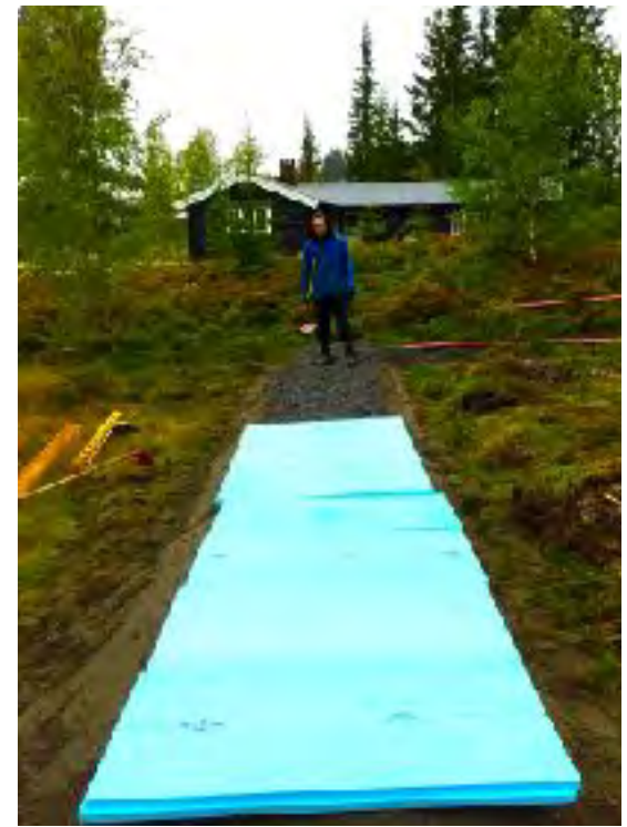
Insulation - 5cm of expanded polystyrene
