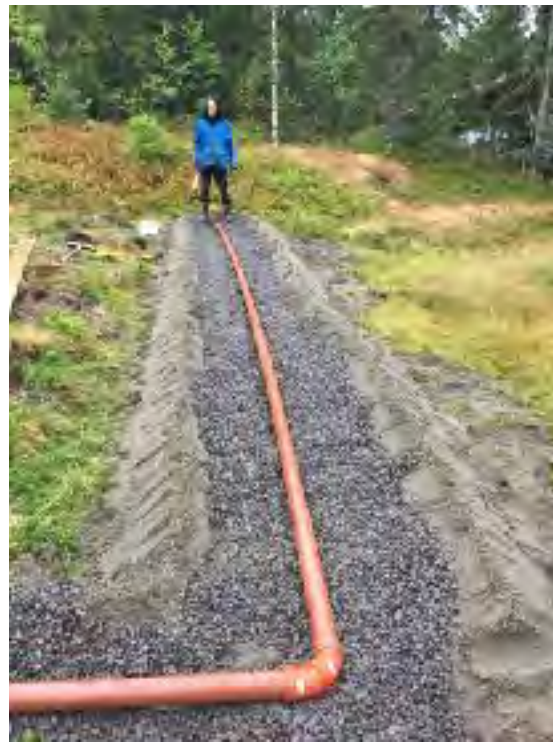
Gravel and distribution pipe in place
