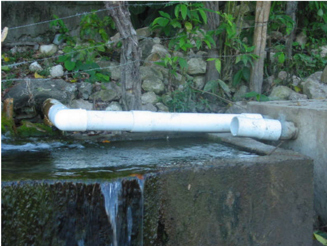
Figure 4.27 Connection to transmission tank
