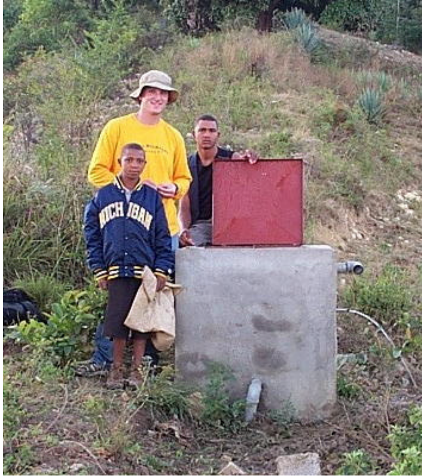
Figure 4.30 Completed Break-Pressure Tank
