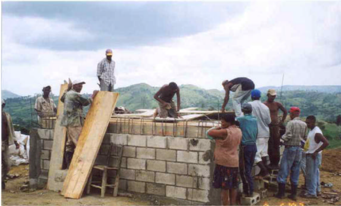
Figure 4.21 Bond beam and false floor construction
