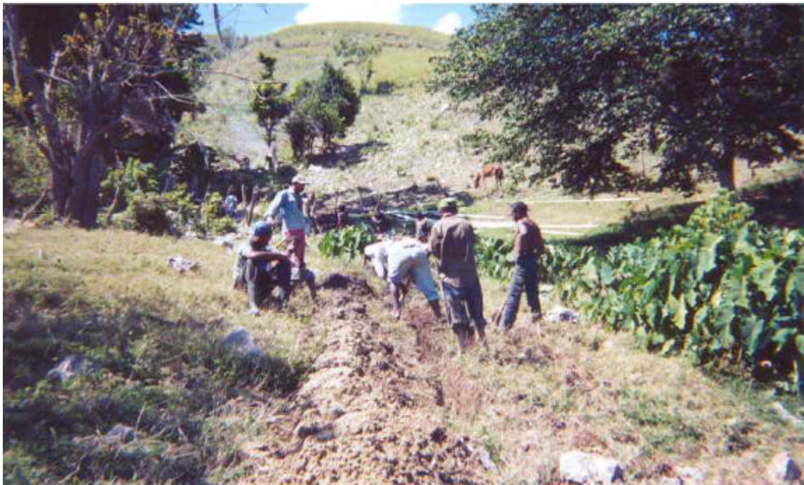
Figure 4.16 Work brigade digging pipeline trench
