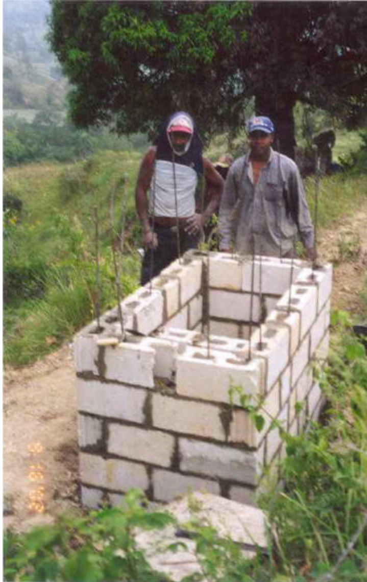
Figure 4.29 Break-Pressure Tank under Construction
