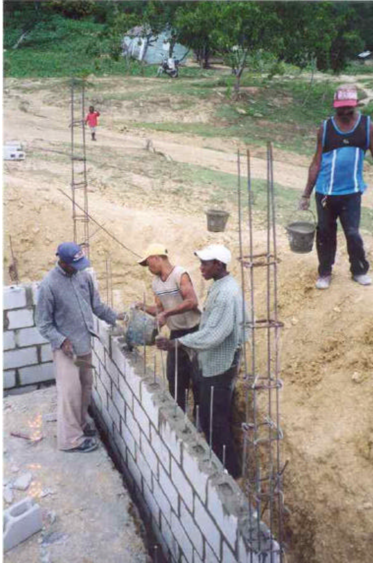
Figure 4.19 Filling in Block Cavities.
