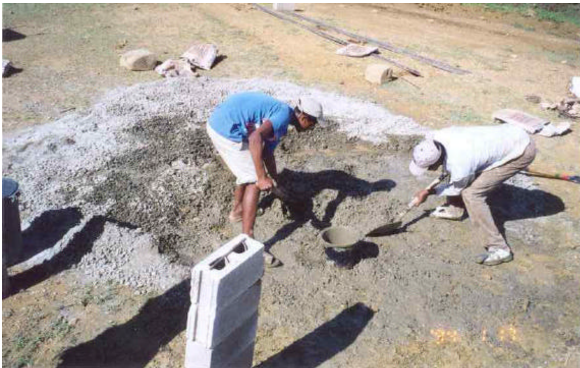
Figure 4.18 Mixing concrete
