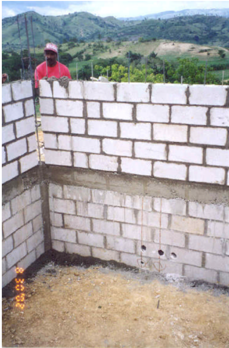
Figure 4.20 Rough interior walls
