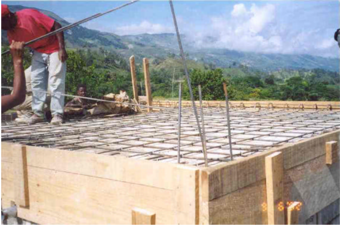
Figure 4.22 Roof rebar preparation
