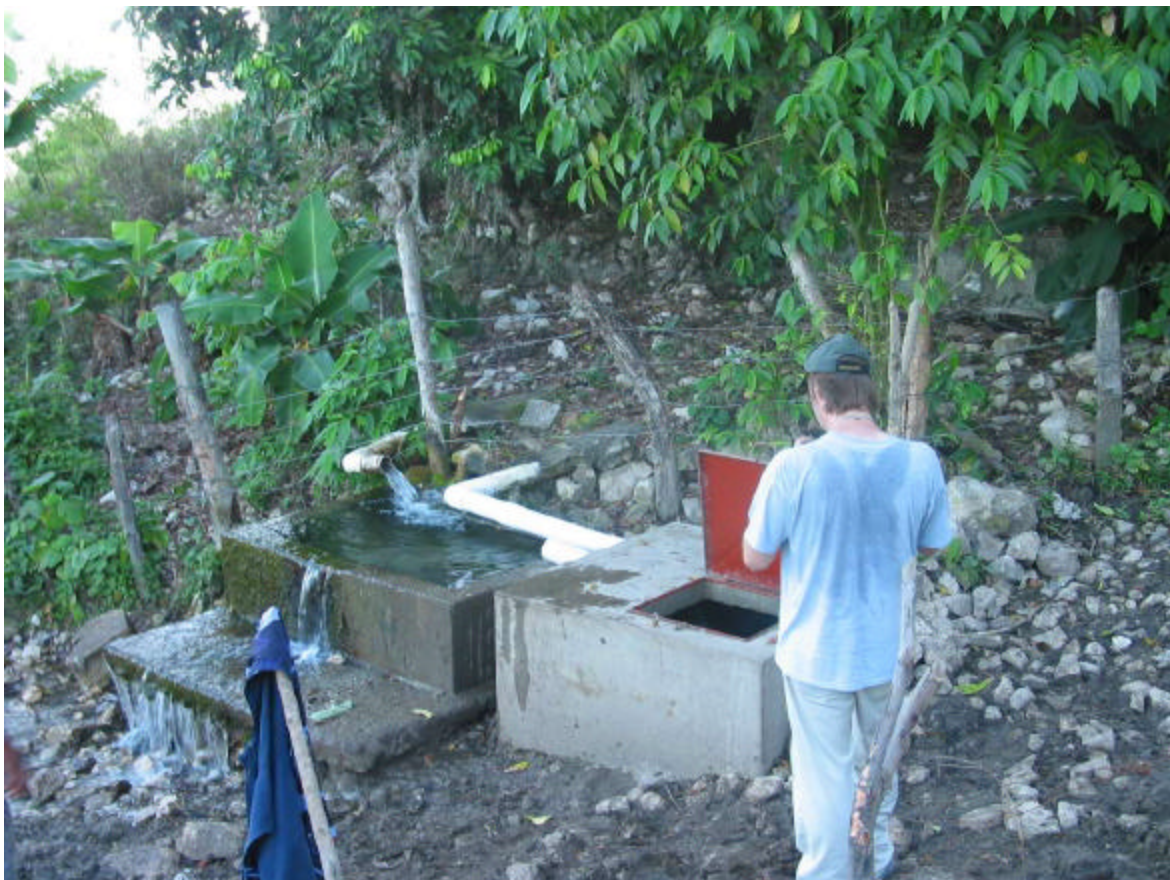
Figure 4.26 New and existing spring construction
