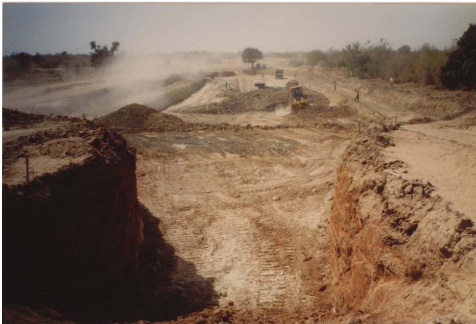
Photo 4.2: Construction of the subsurface dam -2
