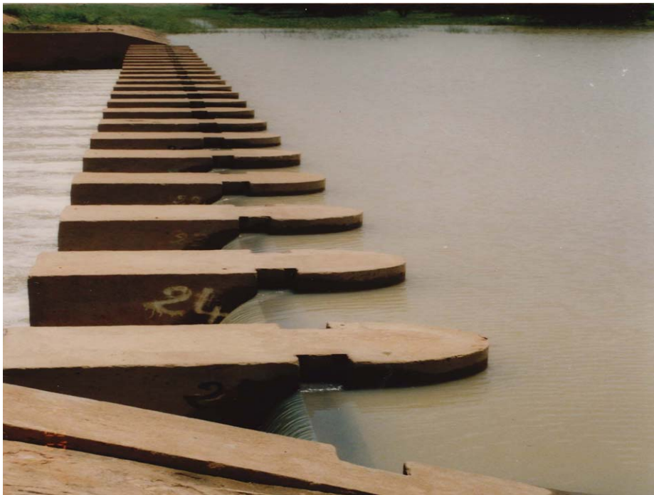
Photo 7.5: Small-scale surface dam with water gates, installed in this project
