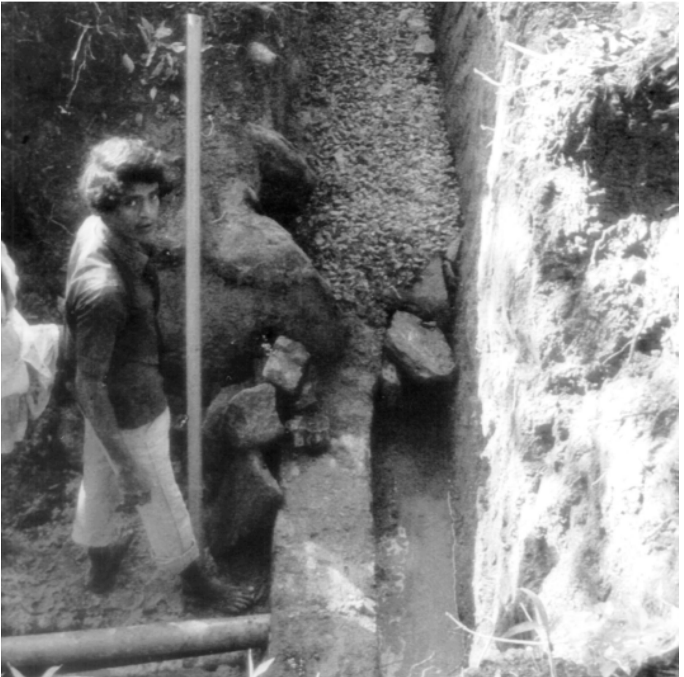
Catchment of contact spring with a "catchment trench"
