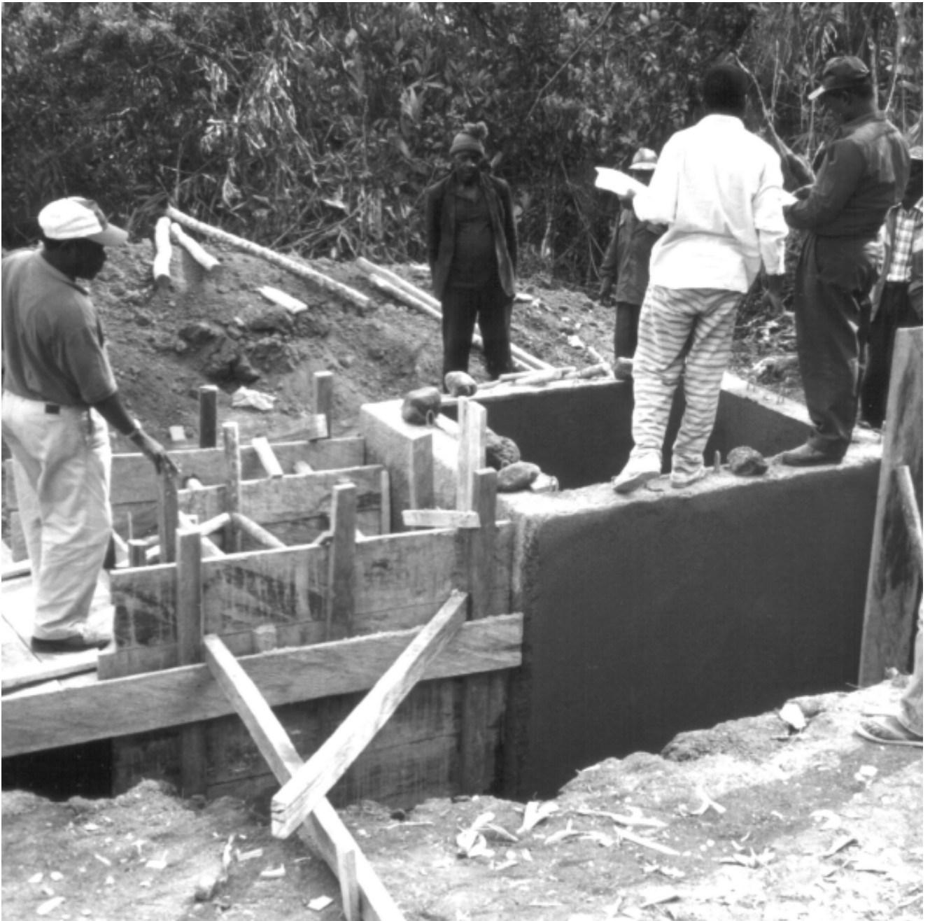
Construction of a spring chamber
