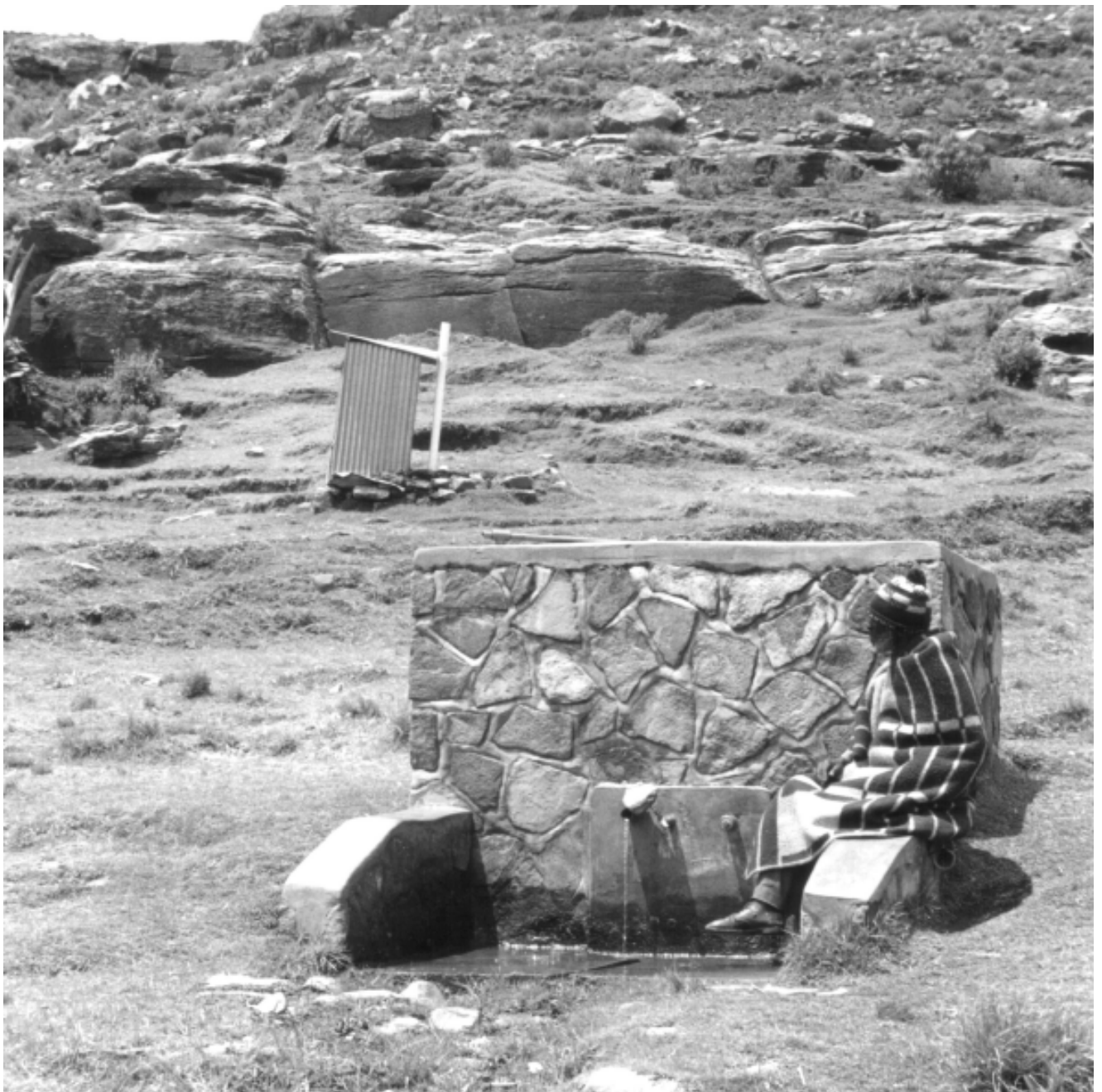
Latrines can be good things but not in the intake area
