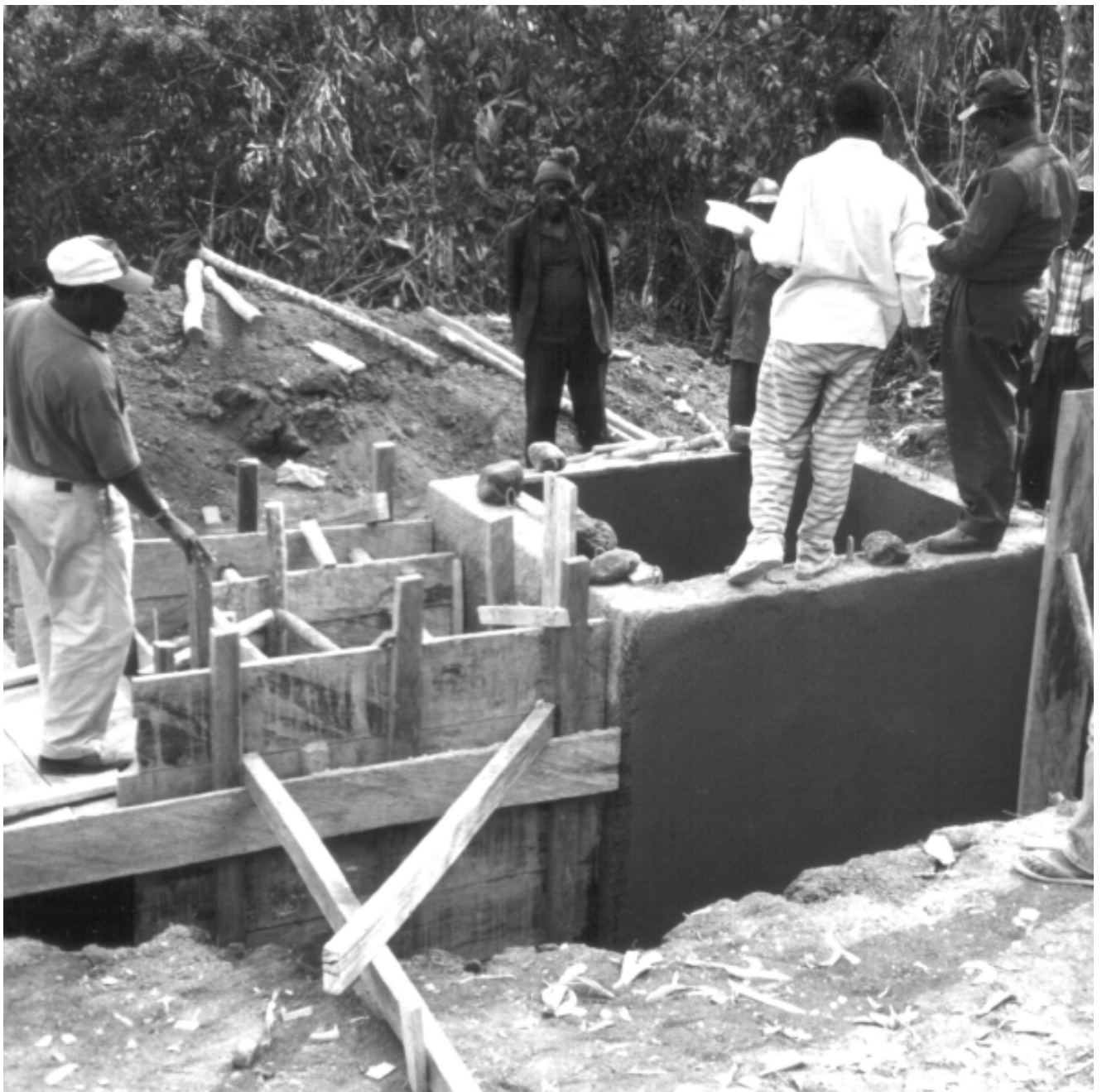
Construction of a spring chamber
