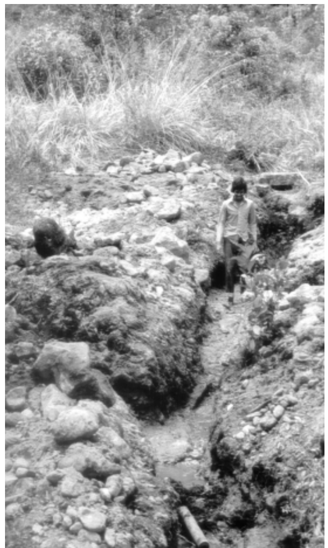
Contact spring with side trench (see Fig. 34)
