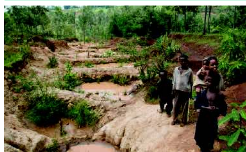
Check dam ponds for gully reclamation on gentle slopes and recharging of groundwater (HP. Liniger)
