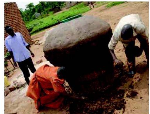
A couple in a Ugandan village building a WH jar at their home. (WaterAid/ Caroline Irby)
