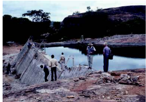
Construction of a rock catchment dam in Kitui, Kenya. (HP. Liniger)
