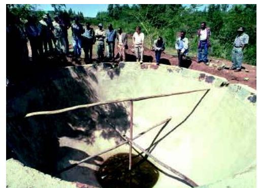
Cement-lined underground tank in construction, Ethiopia. (HP. Liniger)
