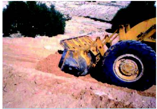
Mechanical construction of a tabia dyke, Tataouine, Tunisia. (M. Ouessar)
