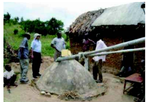
Organic roof with an additional plastic covering and partially below ground tanks in rural Uganda (Danert and Motts, 2009).
