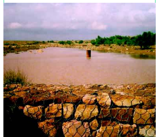
Example of a recharge well behind a gabion check dam after rain. (M. Ouessar).
