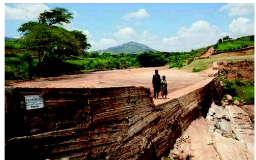
Fully filled sand dam in the Nzyaa Muysio valley in Kenya. (P. Braden)
