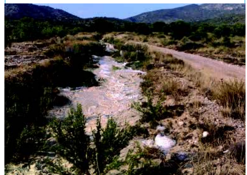
Traditional channel system ( acequia ) directing diverted flood water (by earthen or stone bunds) from intermittent streams towards almond terraces, Spain. (J. de Vente)
