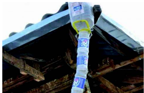
A fallpipe made of old plastic bottles stitched together by thin wire, Tajikistan. (S. Stevenson)
