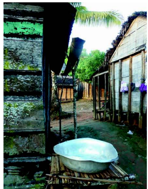
A simple Rooftop WH system supplying drinking water, Madagascar. (J. Zähringer)
