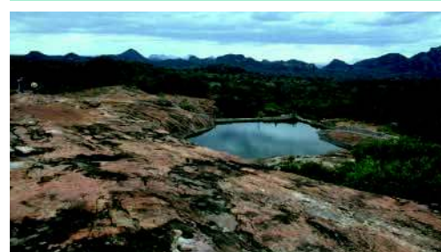
Rock catchment dam in Kitui, Kenya. (HP Liniger)
