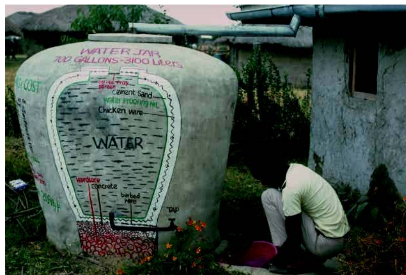
Steps for constructing a cement water tank using a plastic bag filled with straw. Drawing on tank shows design and material needed. (HP. Liniger)
