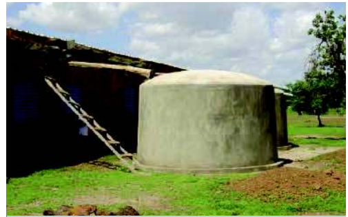
A ferro-cement tank at a local school in Burkina Faso. (WaterAid / Chris Leake)
