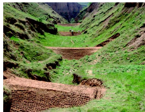
Warping dams in Xifeng county, province of Gansu after establishment of the structures. (L. Xiaobo)
