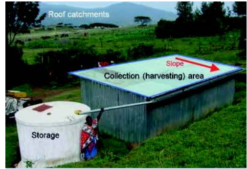
Roof catchment in Kenya showing the different components of a rooftop WH system. (M. Malesu).
