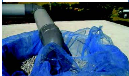
A filter with mesh, sand and gravel used in Karnataka, India (Rainwater Club, not dated).
