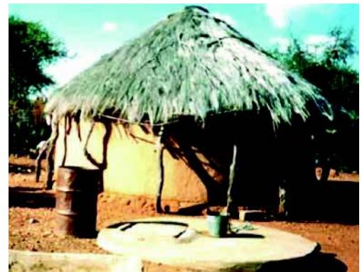
Rooftop WH system with rainwater collected from an organic roof. (www.infonet-biovision.org)
