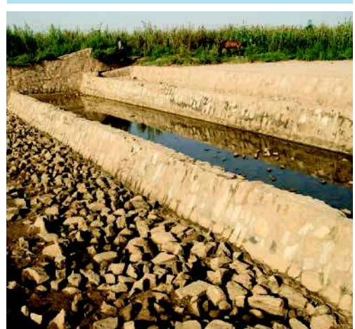
Water spreading weirs built in series (GIZ, 2011).
