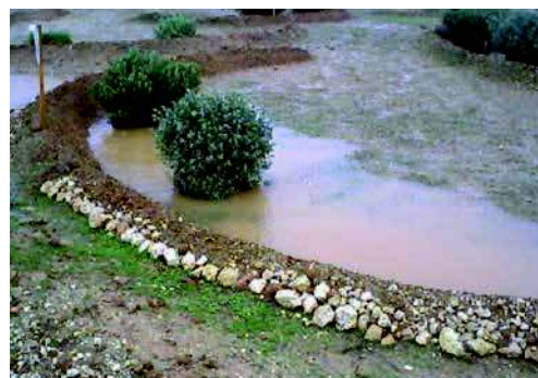
Semicircular bunds with olives collecting water. (T. Oweis)
