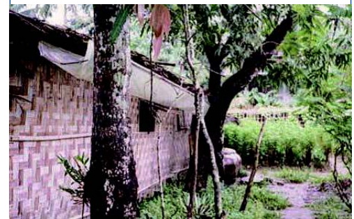
When rain is expected the house owner attaches a wide and removable gutter made of plastic sheet below the roof.
