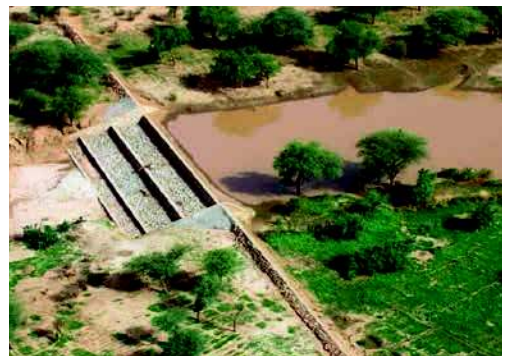
Water spreading weir in the Sahel (GIZ, 2011).
