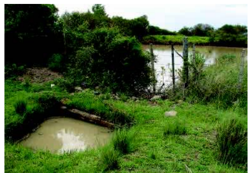
Small earth dam with sedimentation trap in Kenya. (HP. Liniger)
