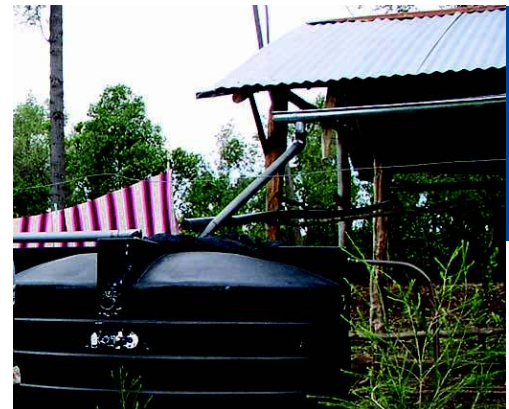
Semi-circular guttering with "circular" extended guttering. (C. Studer)
