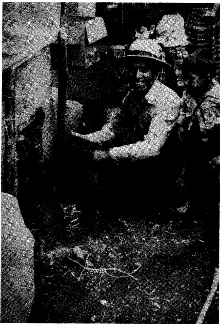
Figure 3.3 A DAFF latrine in Guatemala being emptied The digested excreta is then applied to the land
