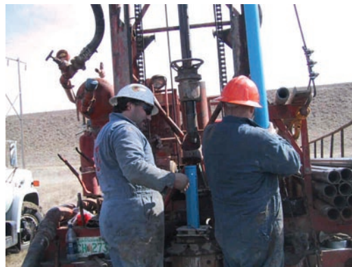
Figure 10: Casing Installation
