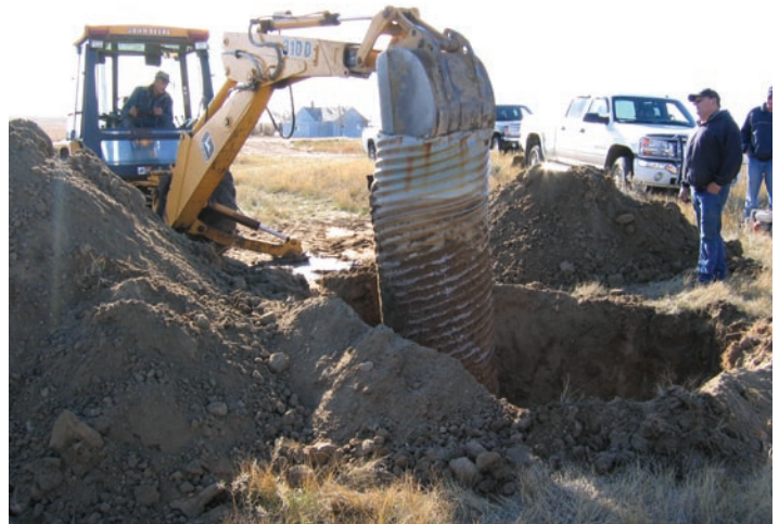
Figure 31: Removal of well casing
