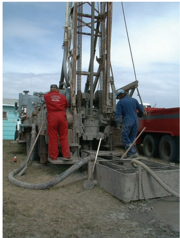
Figure 7: Well Drilling (Courtesy of Agriculture and Agri-Food Canada – Agri-Environment Services Branch)
