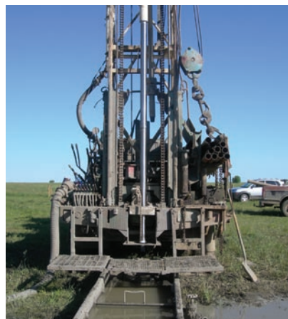
Figure 11: Lowering well screens
