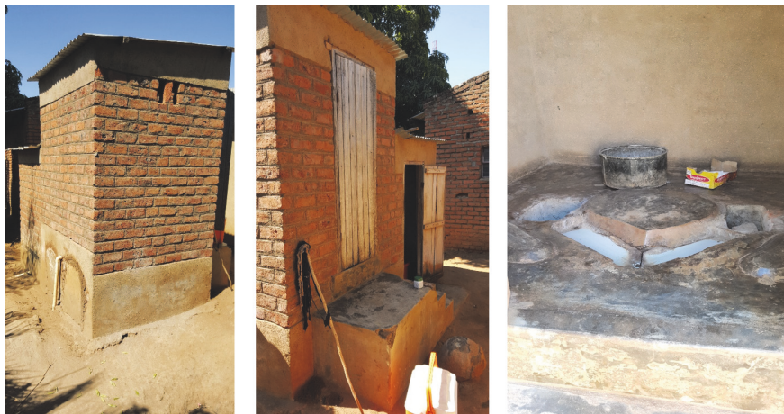
FIGURE 2: UDDT back view, front view, and inside showing urine diverting system and two drop holes, Blantyre, Malawi.
