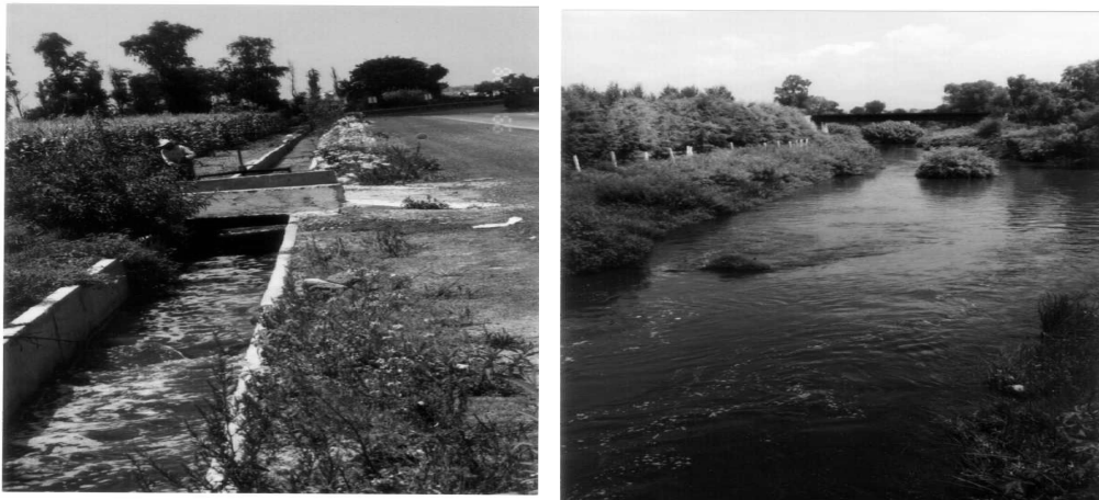
(a) Primary Requena canal near Doxey, lined (b) Secondary canal near Tlaxcoapan, unlined Figure 23.3 Irrigation channels in The Tula Valley.
