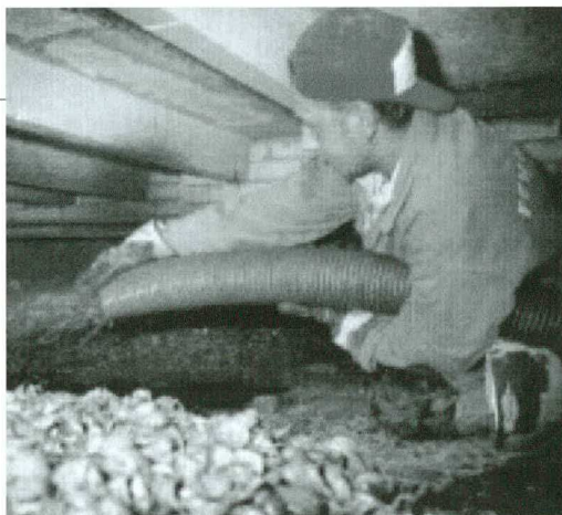
Figure 8.28 Applying the insulating shells
