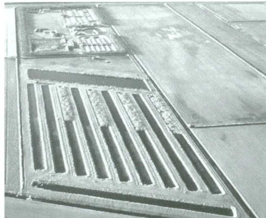
Figure 5.52 Eversteekoog: Areal view of the Eversteekoog constructed wetland, on the background the STP (photo: Simon Smit, Texel)
