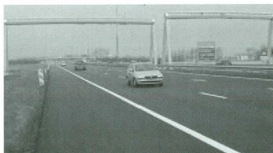
Figure 8.31 Photo of the gantries at Alkmaar
