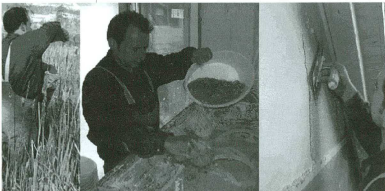
Figure 5.40 Harvesting and using Typha seeds as a additive for clay plaster production
