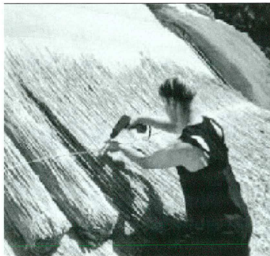
Figure 8.27 Applying a thatched srew roof
