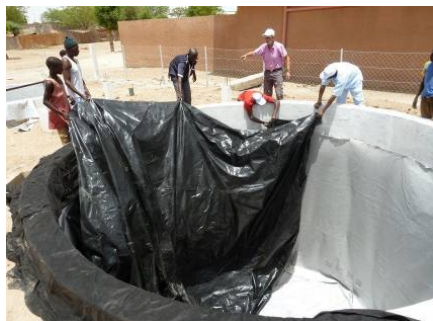
Artistic impression of RainCAP 50m³ and installation of RainCAP system in Senegal
