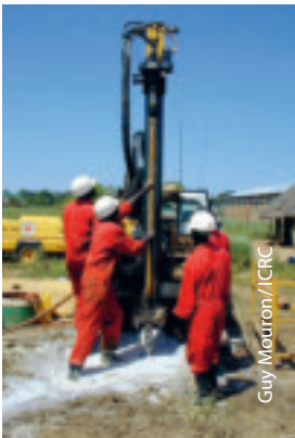
Picture 1: Borehole drilling
