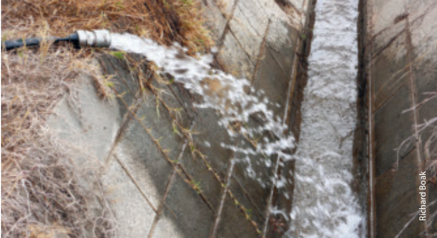
Picture 12: Discharge into surface-water channel
