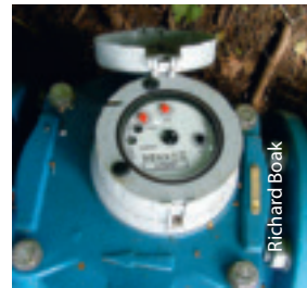
Picture 6: Water meter
