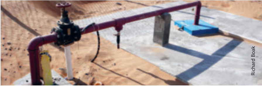
Picture 11: Gate valve in discharge pipe
