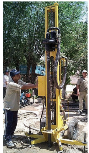
Figure 5: A PAT 301 drilling rig
