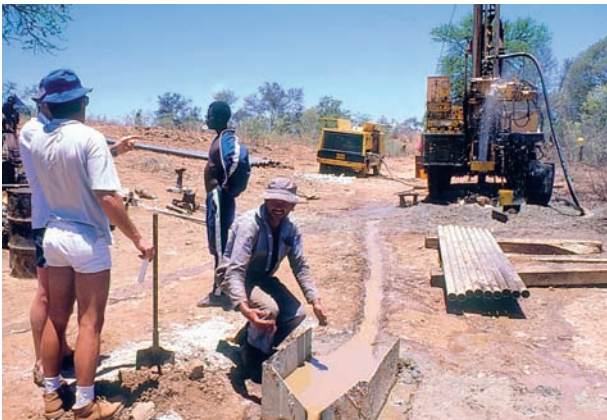
Figure 15: Measuring the blowing yield of a newly drilled borehole
