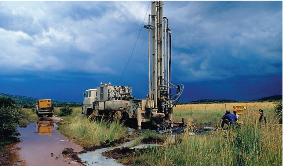
Figure 3: Air rotary machine developing a successful borehole, South Africa, 1989
