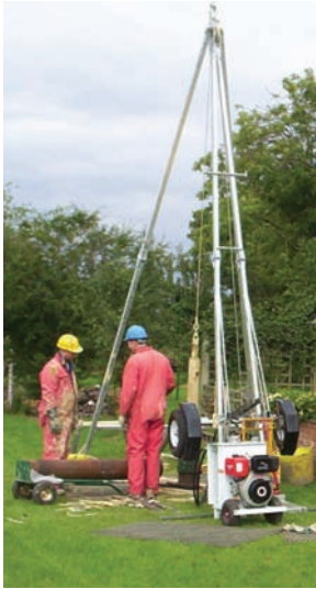
Figure 4: The Forager 55 cable-trailer rig in use
