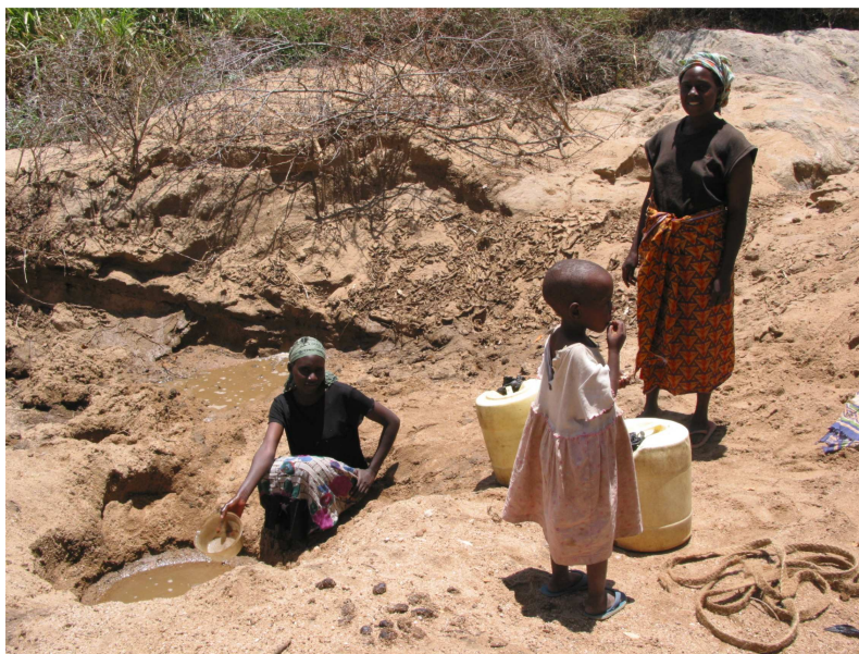
Figure 1.2 Groundwater abstraction from the riverbed by means of a scoop hole (10-10-2006)
