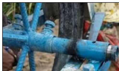
Nuts are welded on the hub pipe
