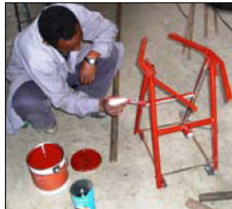
Painting with anti-rust paint
