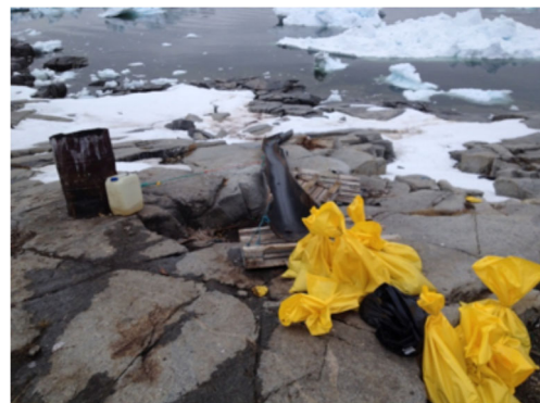
Fig. 2 Local system from a village with about 40 people for discharge of black water from the toilet bags. A local sanitation worker cuts the bags open and pours out the contents. Beside the ramp is a metal bucket for the bags and a bottle with liquid for cleaning
