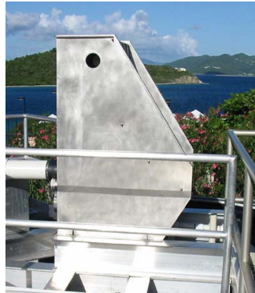
TYPICAL INFLUENT STATIC SCREEN
