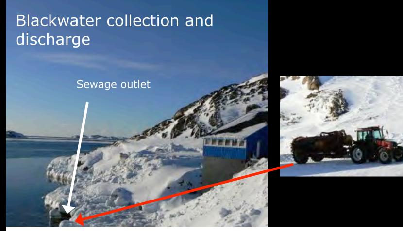
The honey buckets collected with a tractor and a vacuum tank are emptied at the «Chocholate factory» the blue building in the picture. The excreta is discharged untreated.
