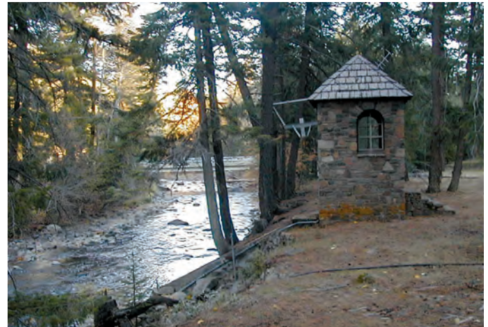
Stream-gaging station on the American River near Nile, WA (USGS Station No. 12488500), one of more than 6,600 across the Nation with real-time streamflow data. (Photo by Van Wilson, USGS.)
