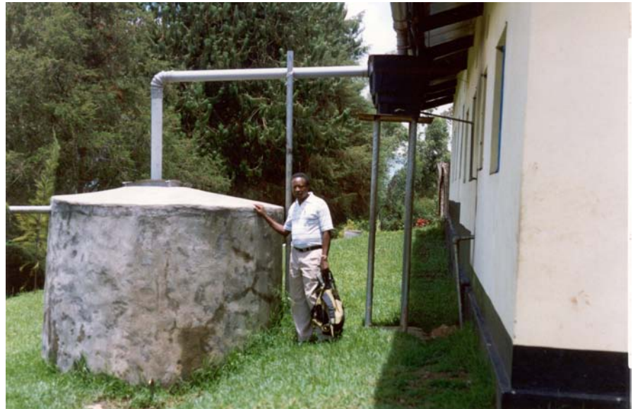
Photo 1: Rainwater harvesting. (Source: WEDC © Brian Skinner)
