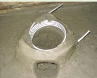
Photo 8: Construction of a flow-through system in a traditional Bangladeshi clay oven. (Source: Richard Johnston, UNICEF in Fakhrul Islam et al., 2006)
