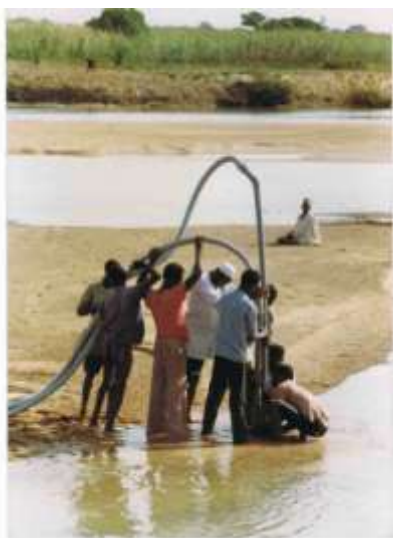
Figure 20. Well Jetting in Action
