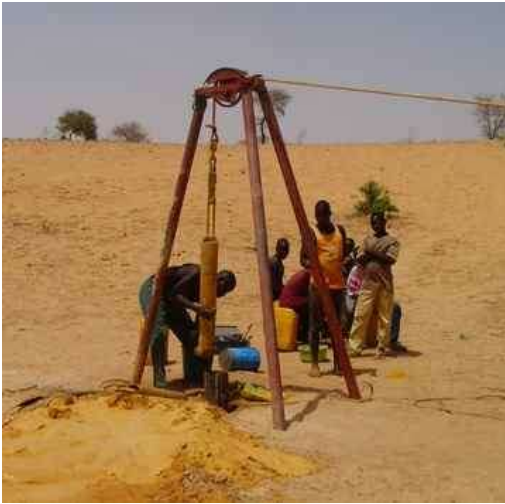
Figure 5. Hand percussion rig in action
