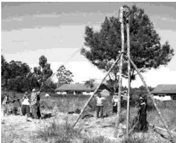
Figure 8. Stonehammer Drilling in Action
