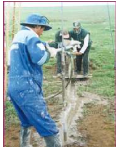
Figure 26. EMAS Drilling
