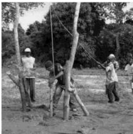
Figure 13. Reaming of a Baptist drilled hole by sludging
