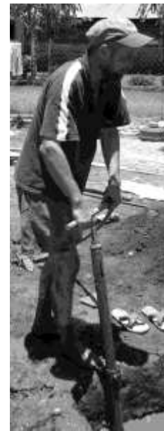
Figure 24. Hand operated mud pump
