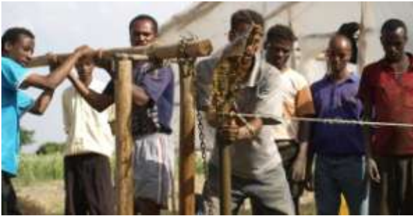
Figure 17. Rota sludge drilling
