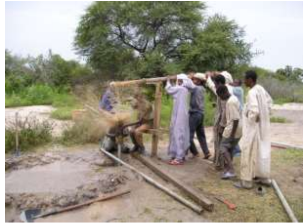
Figure 27. Rota Sludge Drilling
