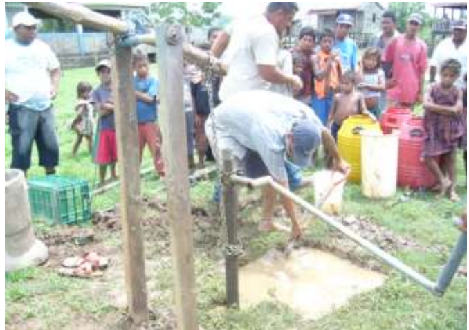
Figure 30. Removing Cuttings from Settling Pit
