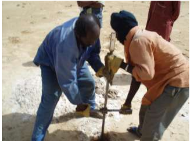
Figure 28. Hand Drilling a Tubewell
