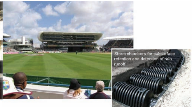
Figure 33 (A) Rainwater capture from a municipal facility in Charlotte Amalie, St. Thomas, USVI; 33(B) Rainwater harvesting for irrigation of Kensington Cricket Oval, St. Michael, Barbados (runoff from field and roof catchments diverted to perimeter sub-surface drain - see inset) (photos courtesy: Henry Smith and Andrew Hutchinson)
