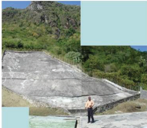
Figure 6 Surface catchment for communal RWH system at Ashton on Union Island, St. Vincent and the Grenadines
