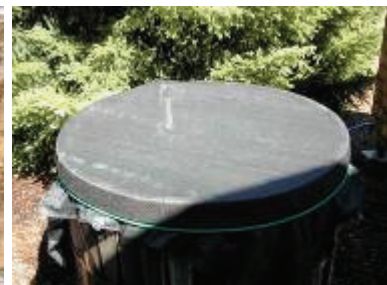
Typical outdoor drum covered with fine mesh (usually for non-potable use)
