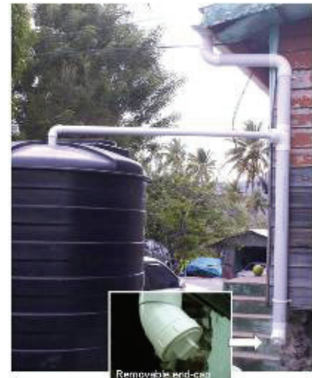
Figure 11 First-flush diverter
