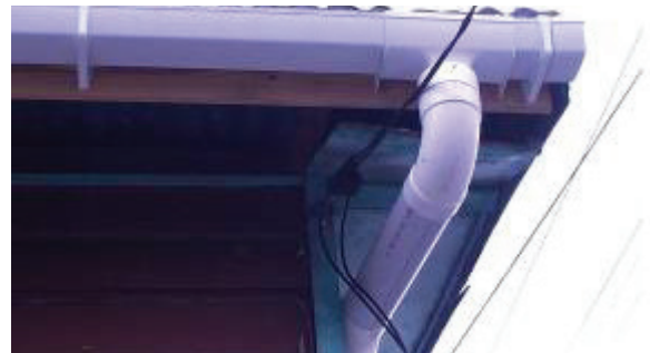
Figure 9 Typical PVC guttering and downpipe
