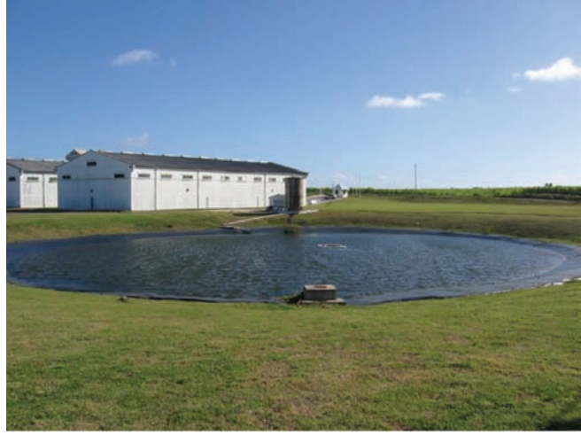
Figure 35 Rainwater harvesting diverted to surface storage at Mount Gay Distilleries, St. Lucy, Barbados; irrigation and firefighting purposes (photo courtesy: Andrew Hutchinson)
