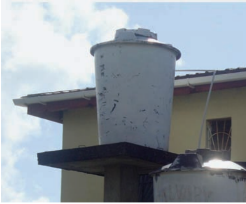
Figure 27: Typical header tank arrangement.
