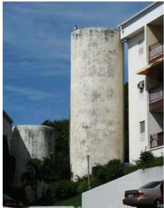
Figure 5 Cistern serving apartment building in St. Thomas, USVI. (Photo courtesy Henry Smith)
