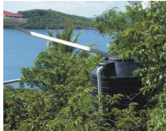
Figure 22 Typical plastic tanks for household RWH system
