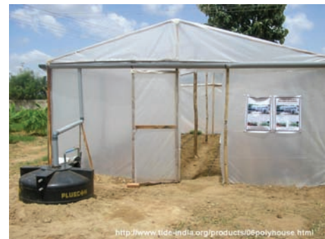
Figure 34 Rainwater harvesting off a greenhouse for irrigation purpose (source: Technology Informatics Design Endeavour (TIDE) http://www.tide-india.org/products/06polyhouse.html )
