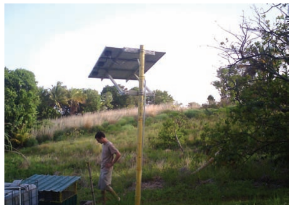
Figure 28: Solar powered irrigation (from surface RWH catchment)
