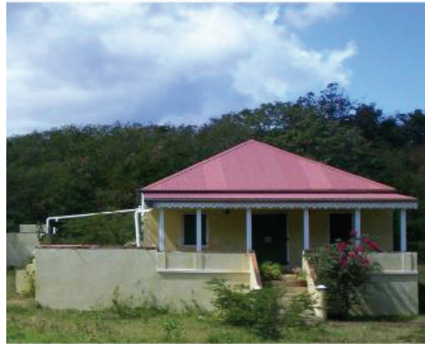
Figure 4 Domestic RWH system with cistern in St. Thomas (Source: H. Solomon and H. Smith, University of the Virgin Islands)
