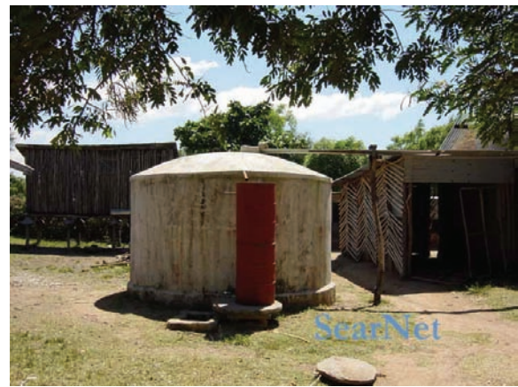
Figure 19 Typical ferrocement tank (source: SearNet – Southern and East Africa Rainwater Network http://www.searnet.org/photogallery/pics/searnetDSC00726.jpg )
