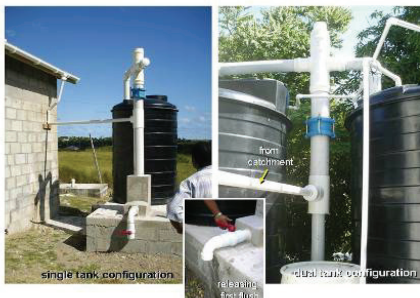
Figure 14 Examples of up-flow filter first-flush diverters (single and dual tank configurations). Used in UNEP/CEHI RWH Project Antigua and Barbuda
