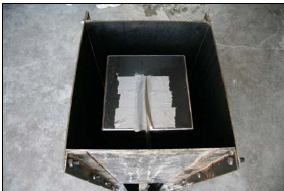
Tape the plastic tubing half way across the interior mold to prevent it from moving and filling with concrete
