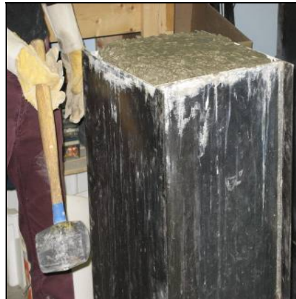
Step 8 - Vibrate the mold with a rubber mallet to help the air escape
