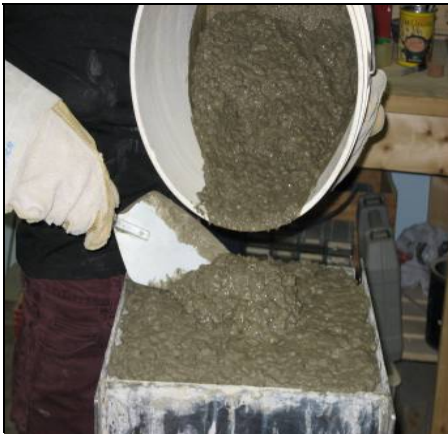
Step 7 - Fill the mold full of concrete
