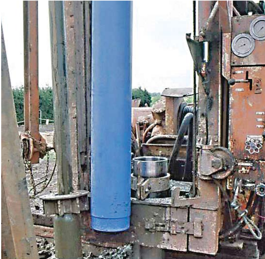
The unit cost of a PVC well casing such as the one shown can be up to 50 percent less than a steel casing
