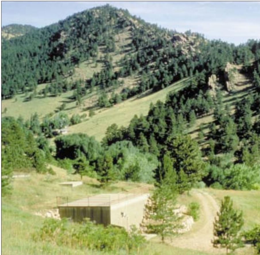
The visual impact of the hydro installations in the Rocky Mountains is minimal.
