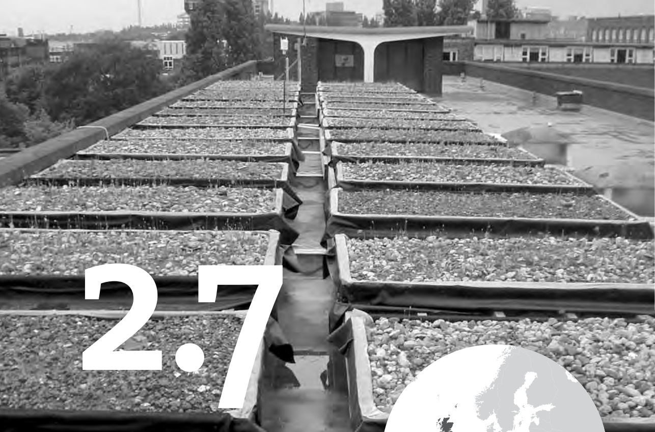
Newly constructed brown roof experimental plots at the University of Birmingham. (Photo credit: Adam Bates)
