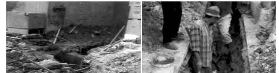
Figure 2.6.4 Excavation in the narrow inner streets of Ma'awa El-Sayadeen
