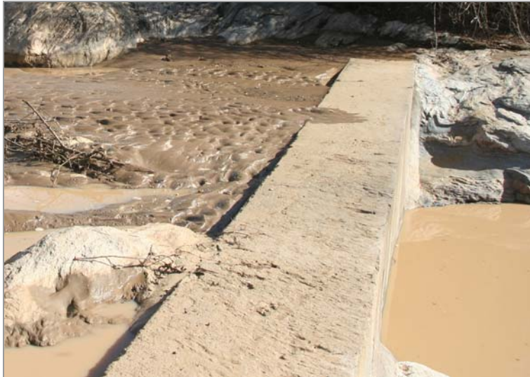
Figure 5.2 Sediment flowing over a dam
