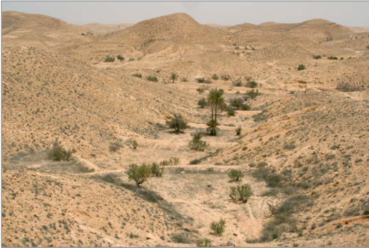
Figure 2.24 Sand storage dams in Tunisia
