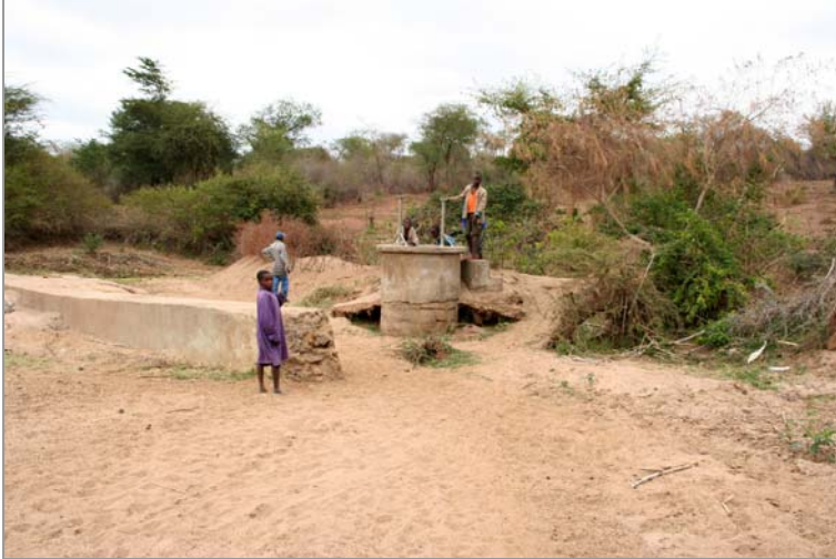
Figure 4.6 Change of river path next to a dam
