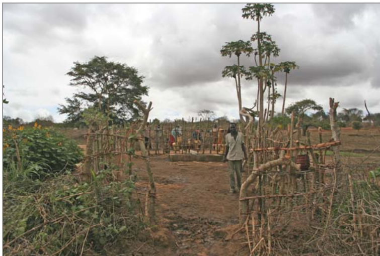
Figure 7.1 A closed well built by AMREF in the Kitui district with a proper fencing to restrict the access of animals to the well
