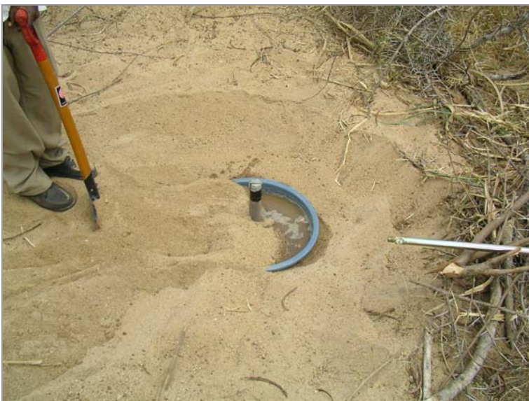
Figure 3.3 Sub-surface evaporation pan during installation
