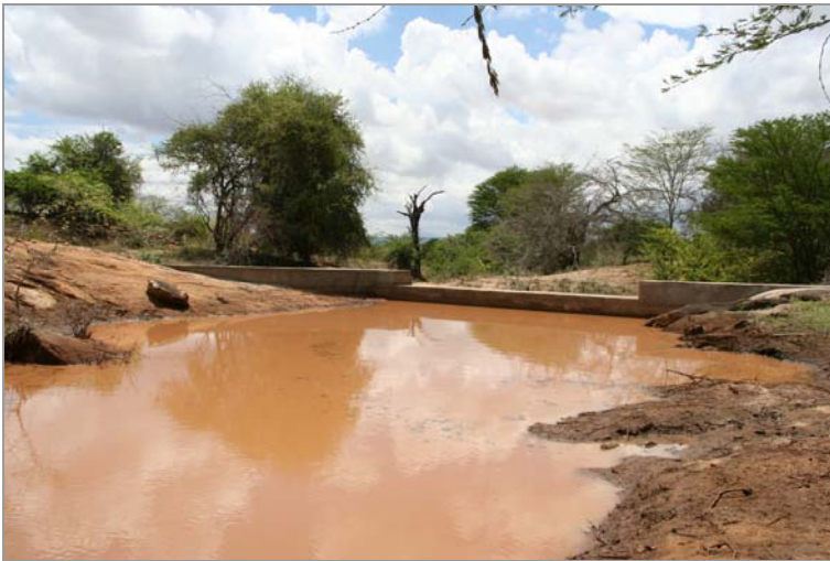
Figure 5.1 Surface water pool behind a recently constructed dam
