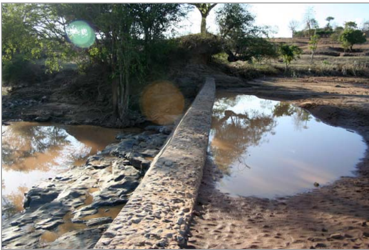
Figure 4.22 Waterlevel up- and downstream of a dam at ground level; the dam is approximately 2.5 m high
