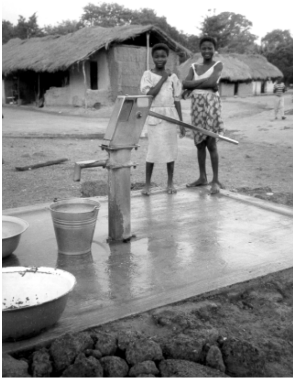
Figure 24 Deep Well Pump
