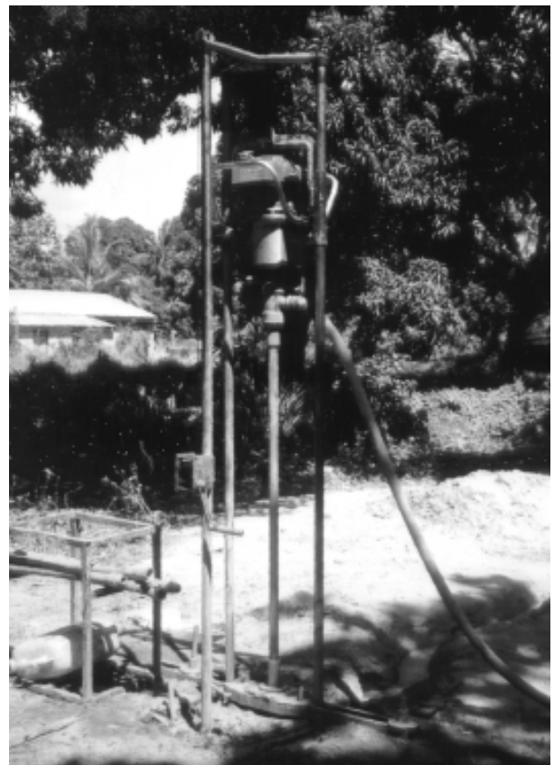
Figure 18 Small Rotary Drill
