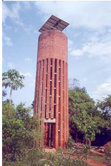
Storage tank in Grace community, Auroville
