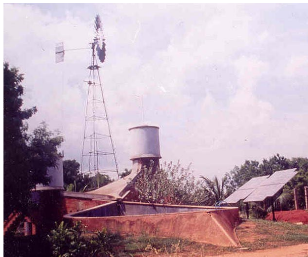
The combined installation in Vikas community
