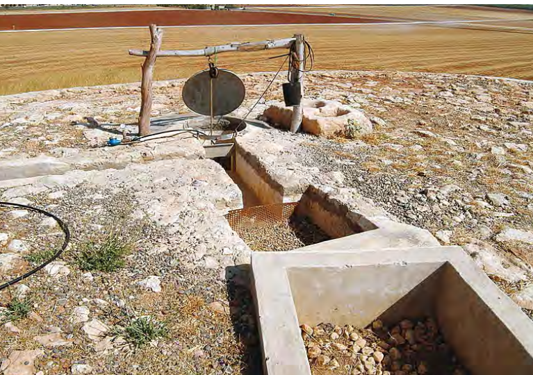
Well designed cistern, with settling basin and sediment trap.
