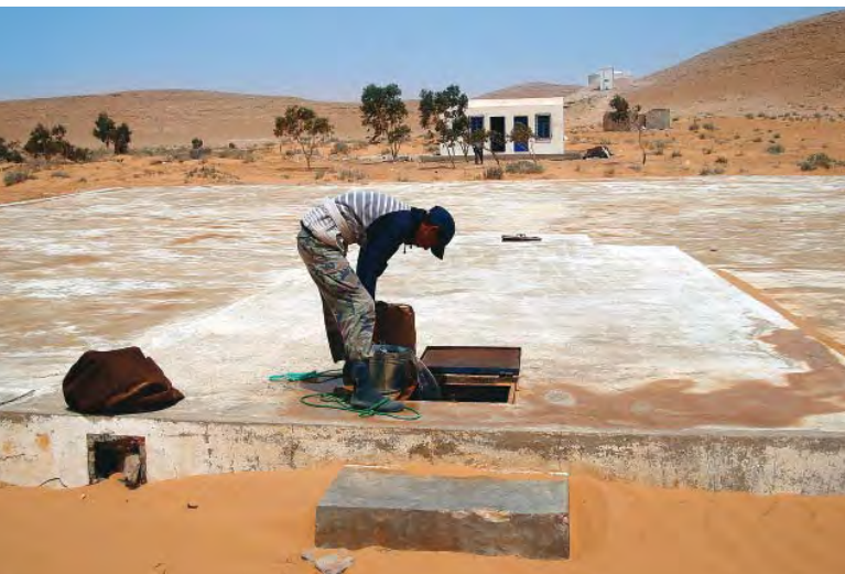
Large numbers of cisterns have been built in the Matrouh region in the past decade, improving local water availability, but also affecting supplies downstream.
