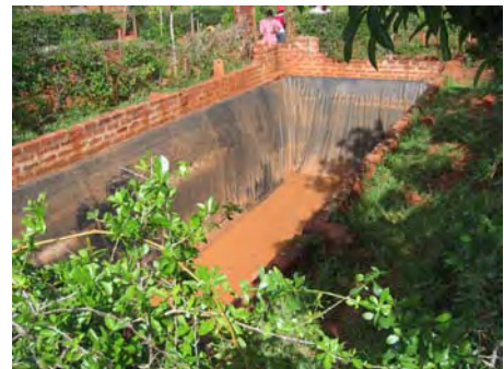
Constructed reservoir to capture runoff near Makutano, Kenya
