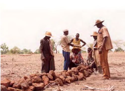
Contour stone bunds constructed and after 2 yrs, Kadiogo, Burkina Faso
