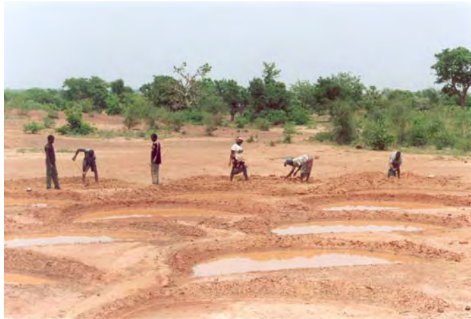
Demi-lunes implementation in Burkina Faso (photo from PDRDP-B/K)
