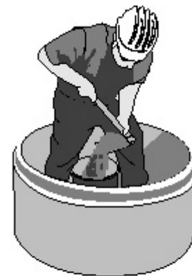
Filling Bucket with Digging Hoe
